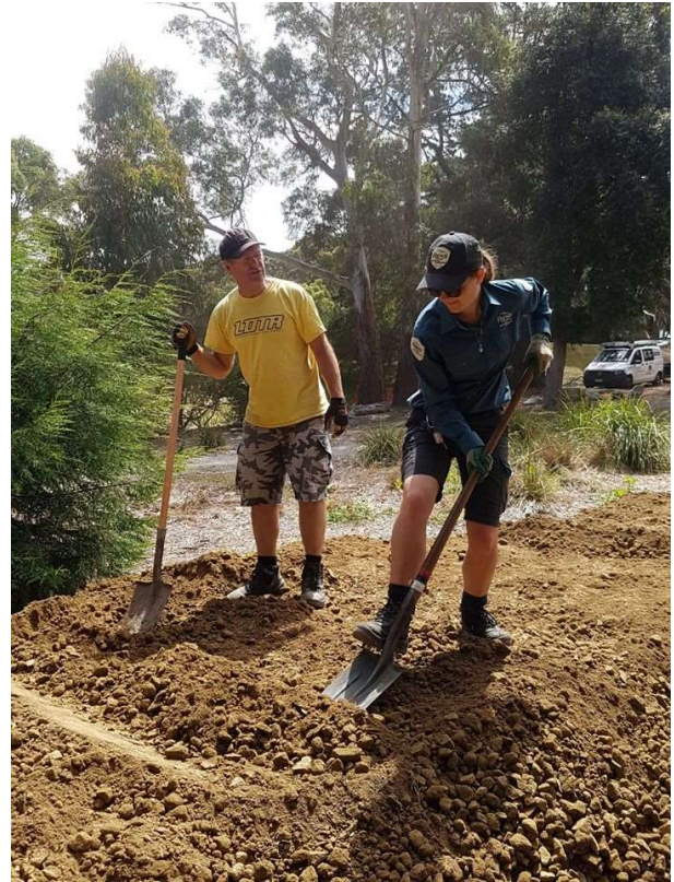
Lysterfield District Trail Riders Trail Build Day
