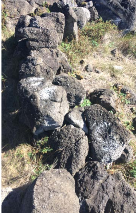
Foundation of stone structure
