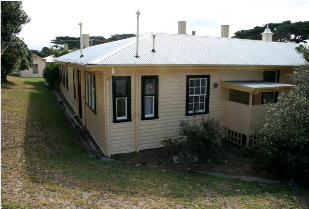
Figure 38 Building 9, southeast view.
