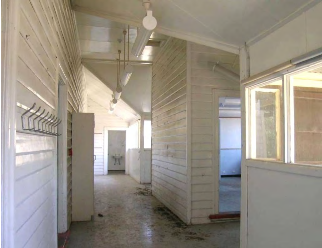
Figure 165 Building 65, looking south along the axis of the former open corridor. The kitchen is to the right.
