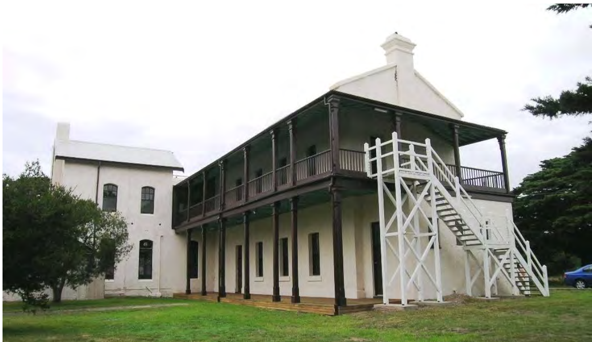
Figure 97 Building 25, northwest view showing the annexe appended to the centre of the building's north façade.
