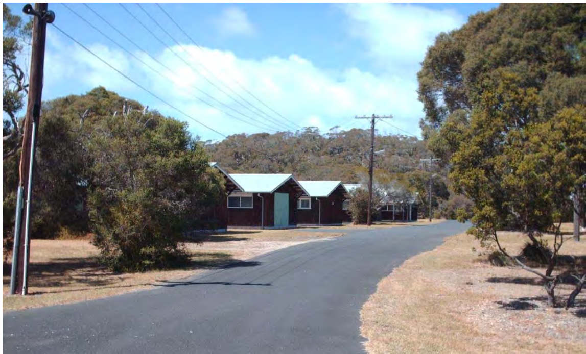
Figure 115 View of the influenza emergency huts, looking south along the access road.
