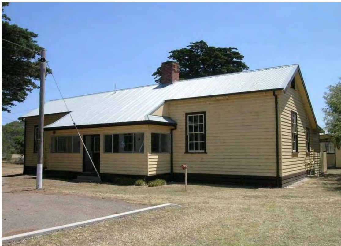
Figure 162 Building 65, showing the east (façade) and north elevation.
