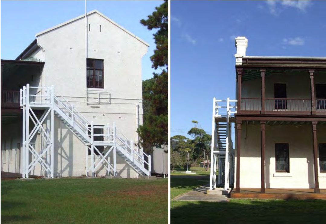
Figure 88 Building 22, from left: west elevation; eastern end of the north elevation.
