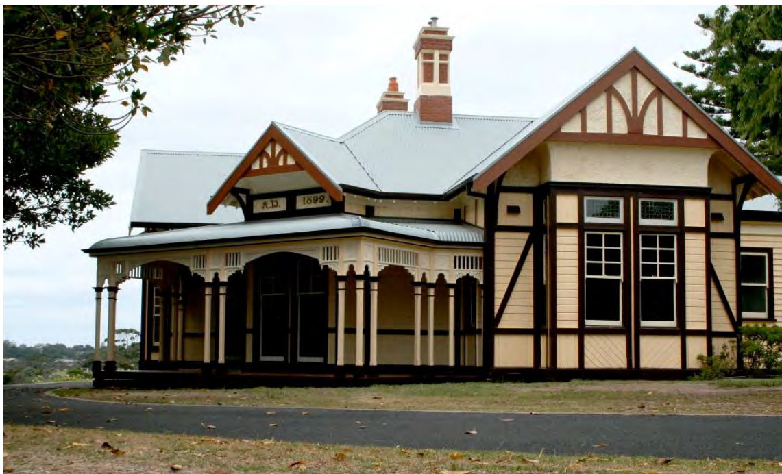
Figure 204 Building 1038, northwest elevation.
