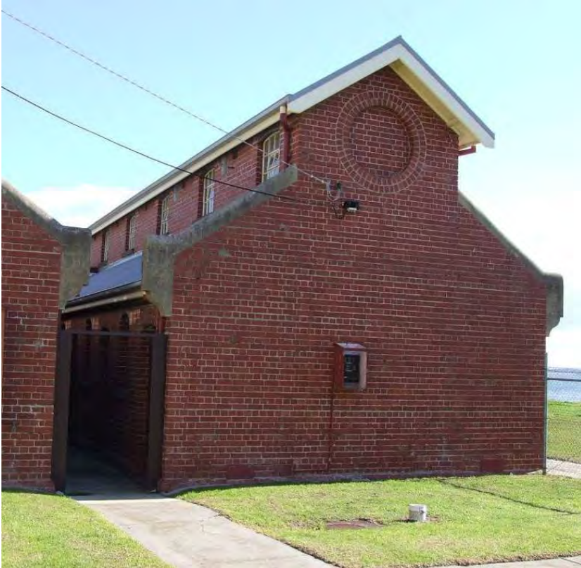
Figure 151 Building 63, view of the east façade.
