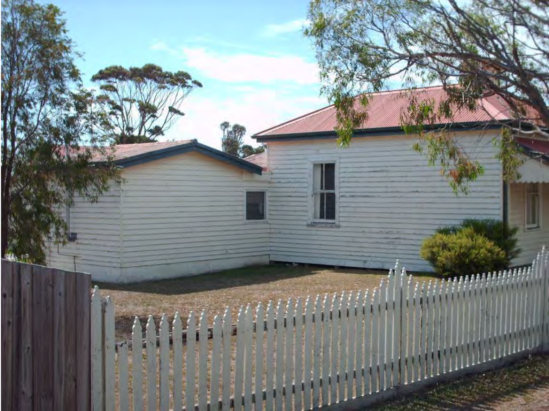
Figure 214 Building 1040, showing the south and west elevations.
