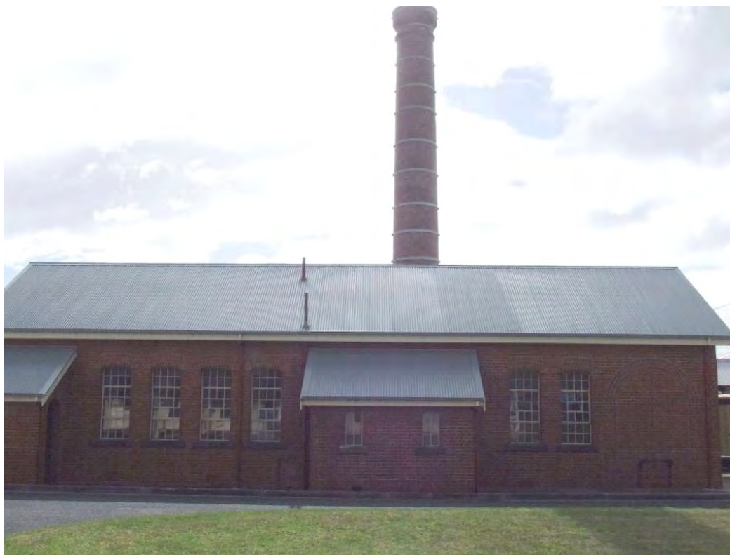
Figure 180 Building 84, south elevation.
