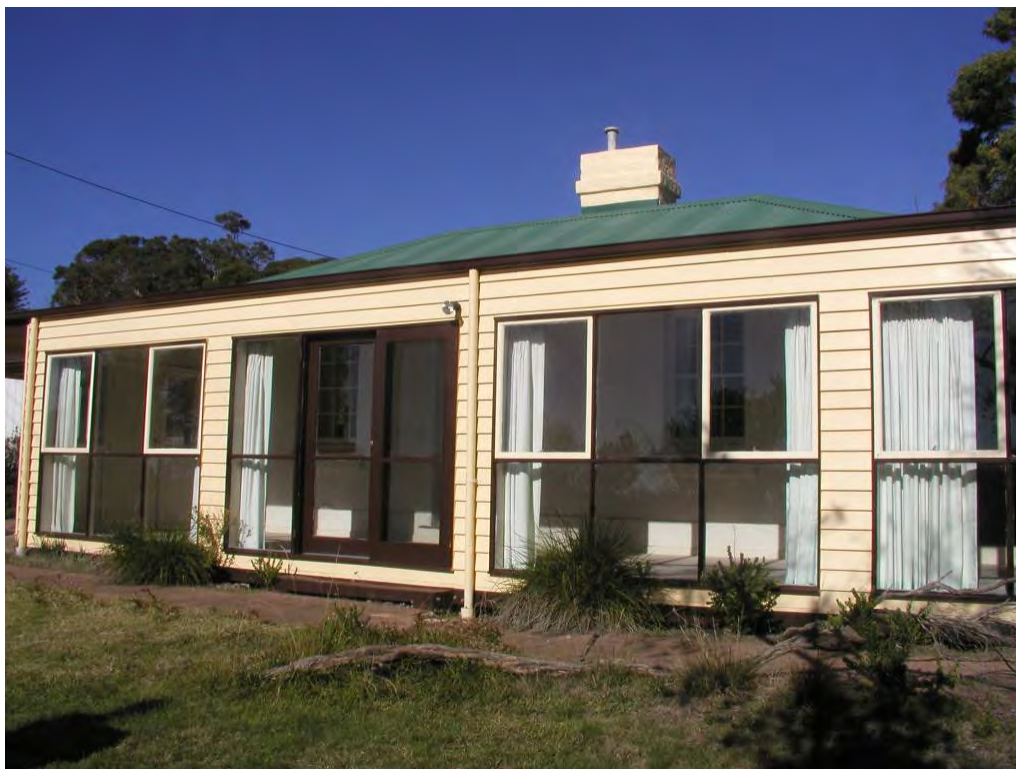
Figure 198 Building 1035, façade. Note the earlier cottage façade, visible behind.
