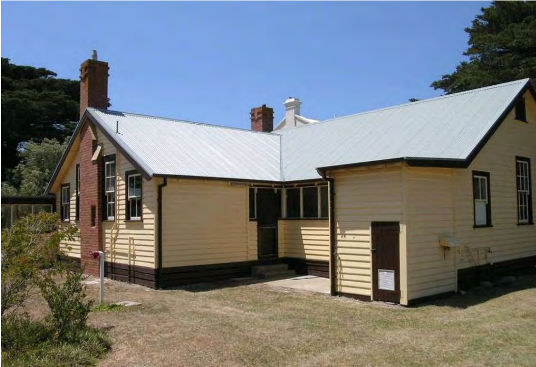
Figure 163 Building 65, showing the west elevation and part of the south elevation.
