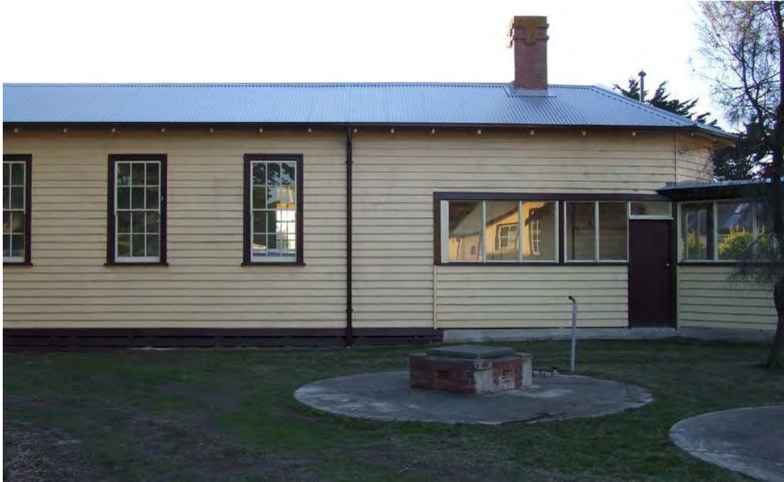
Figure 171 Building 66, showing one of the two isolation wards. The covered walkway – at right – originally joined an open verandah, later enclosed.
