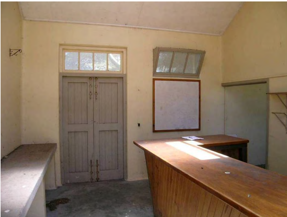
Figure 178 Building 67, interior of the former mortuary. The mortuary slab to the west wall has been retained in-situ.
