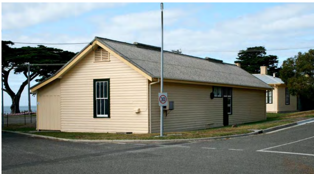
Figure 56 Building 11, southwest view.
