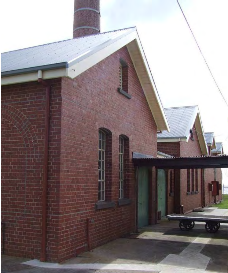
Figure 181 Building 84, east elevation. Note the tram trolley used for the transfer of infected luggage from Building 61 (to right side of picture) to the subject building. The bath houses (Buildings 63 and 64) are in the background.
