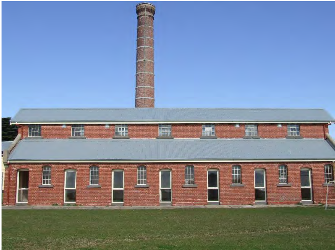
Figure 150 Building 63, north elevation. The chimney in background is associated with Building 84, the Disinfection Building.
