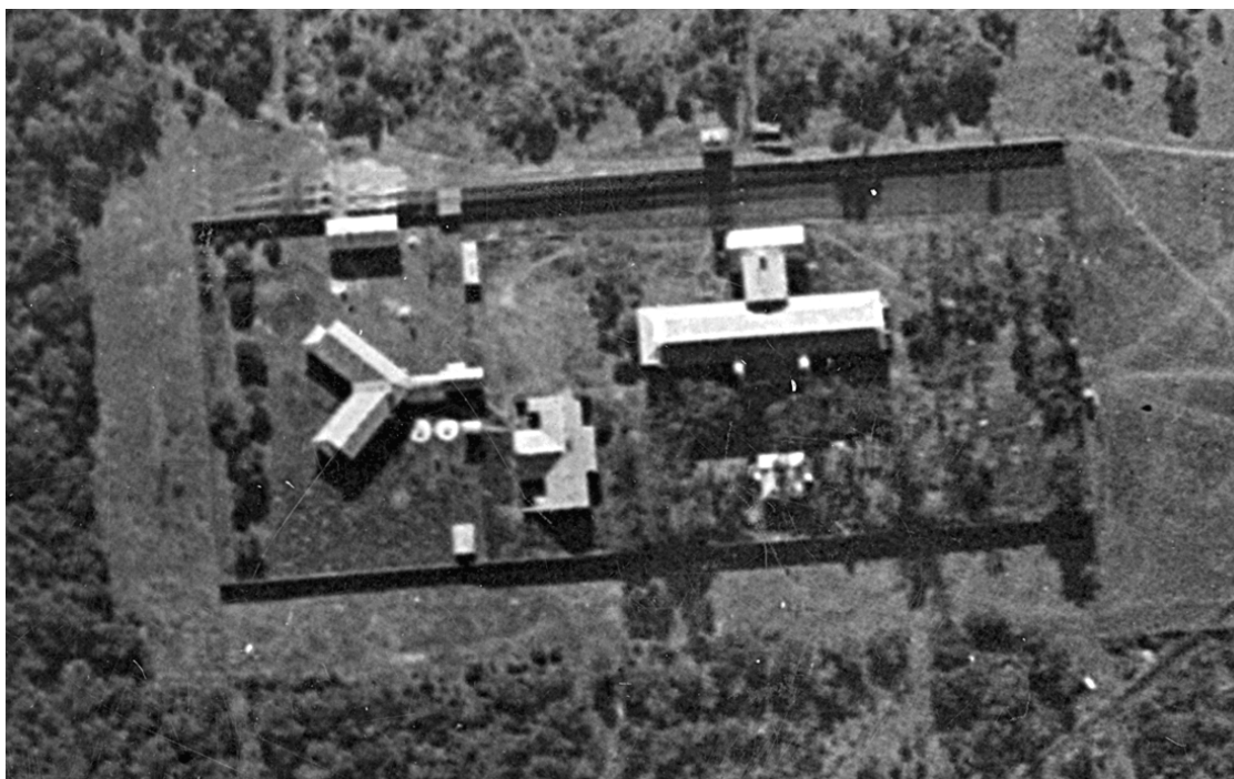
Figure 173 Detail from the c.1922 aerial showing the Isolation Compound, enclosed by a high corrugated iron fence. Building 66 is at left.
