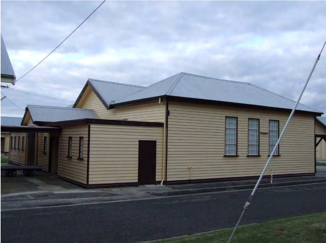
Figure 142 Building 61, showing the south and portion of the west elevation. The building is linked by a covered way to Building 84.
