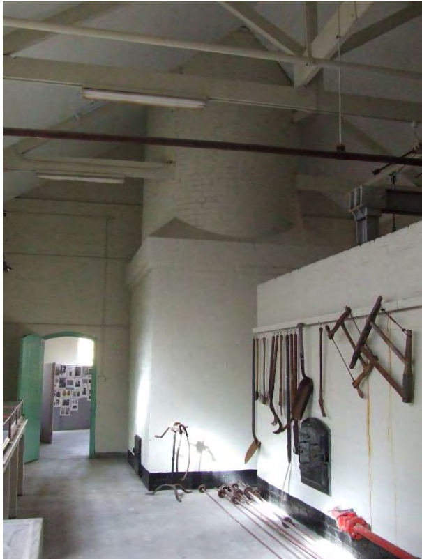
Figure 185 Building 84, interior showing the base of the chimney and part of the museum display.
