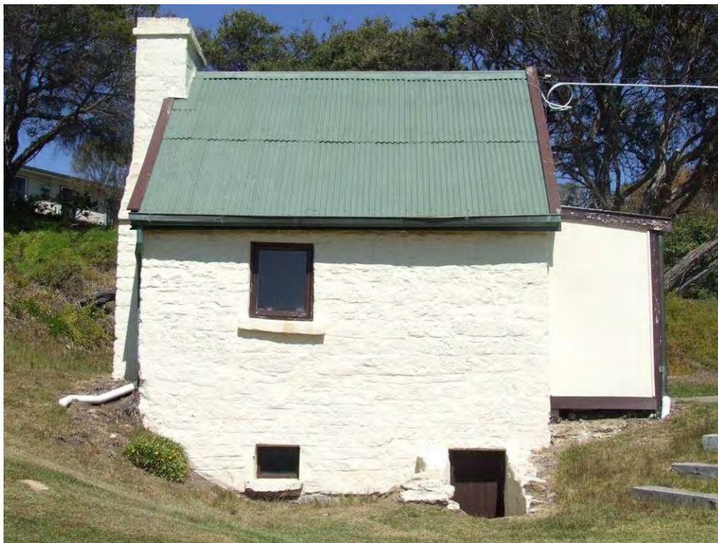
Figure 28 Building 7, north façade.
