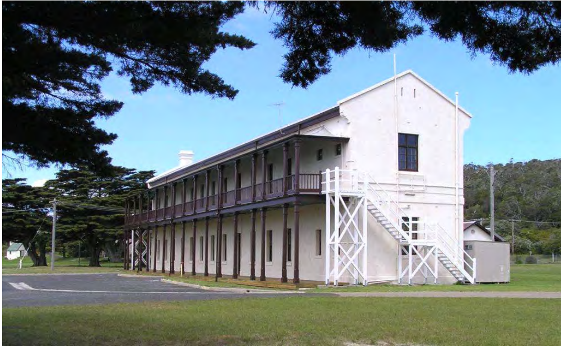
Figure 70 Building 16, viewed from the west, showing the west and north facades. Building 7 is to the left in the distance.
