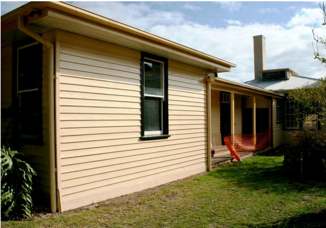
Figure 39 Building 9, view of north façade.
