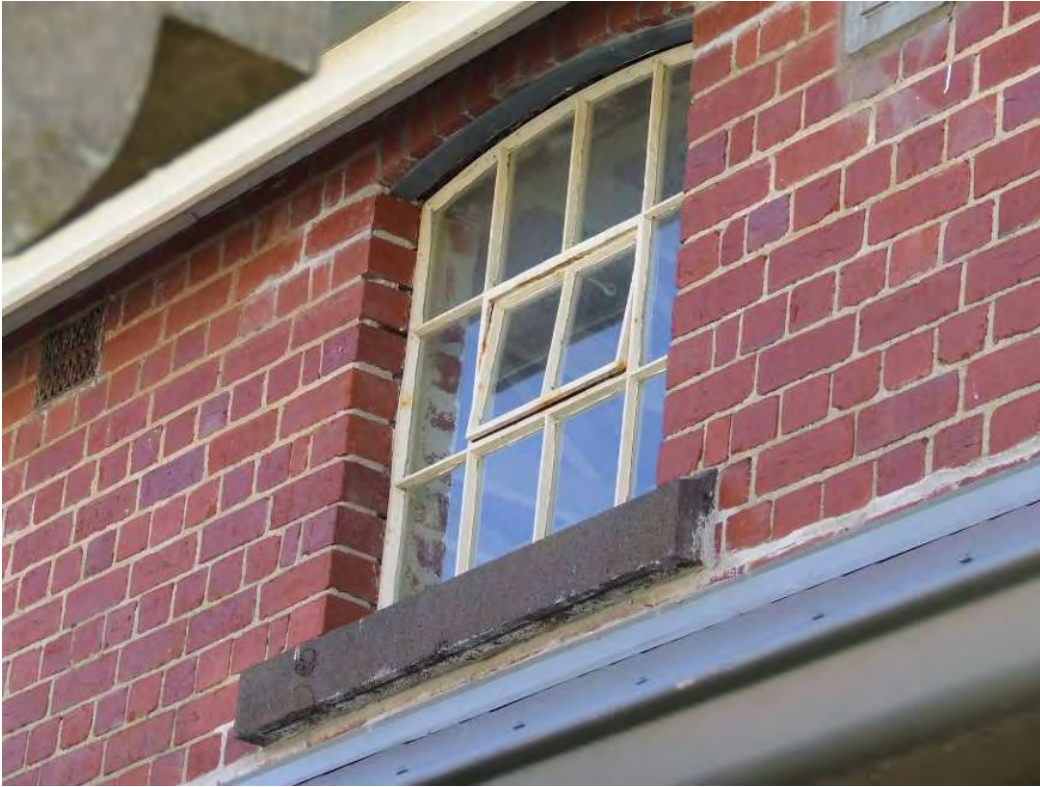
Figure 155 Building 63, showing one of the steel-framed clerestory windows with openable central element.
