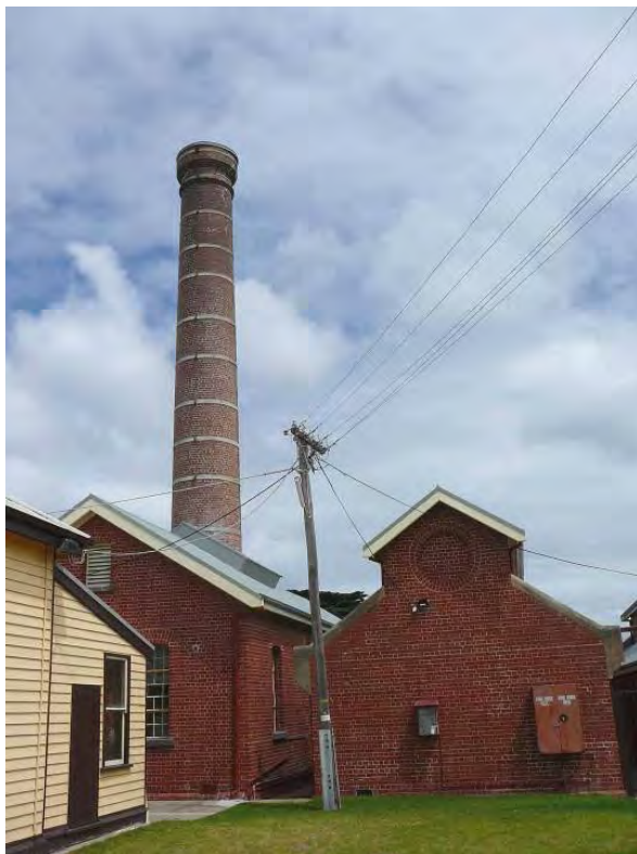
Figure 158 Building 64, showing the east elevation. Building 84 is adjacent (left) and a portion of Building 61 is in the left foreground.
