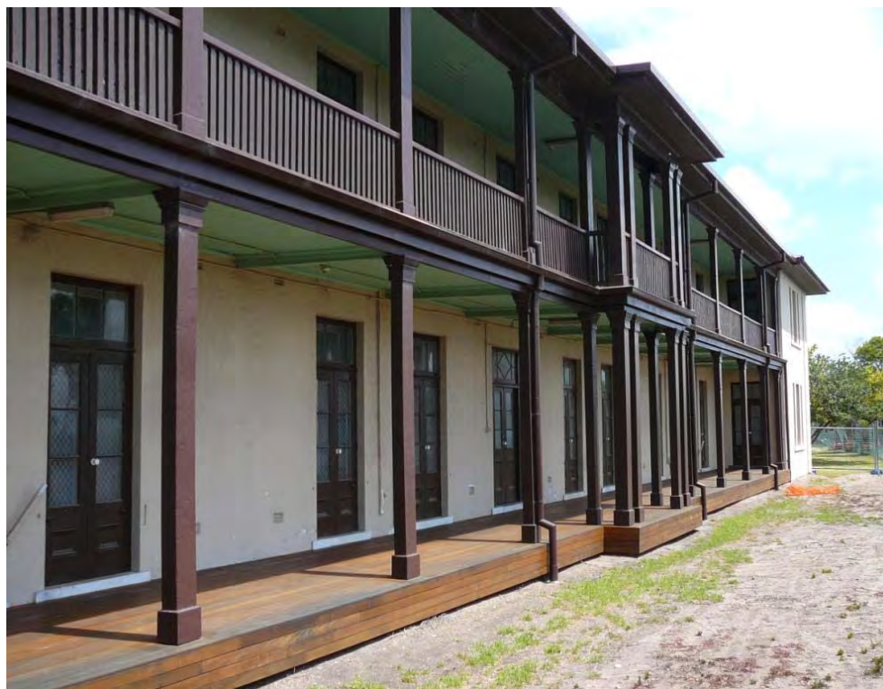
Figure 1 Building 1, partial view of north façade.
