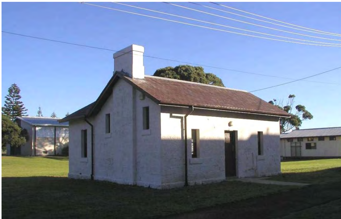
Figure 65 Building 15, showing the north façade with entrance, and gabled east façade with chimney.
