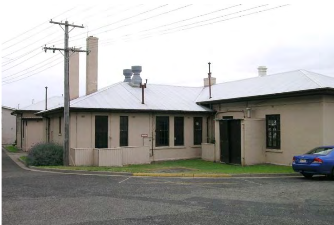
Figure 11 Building 3, southeast view, prior to completion of restoration works.
