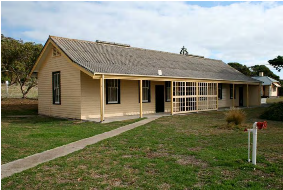
Figure 55 Building 11, northeast view
