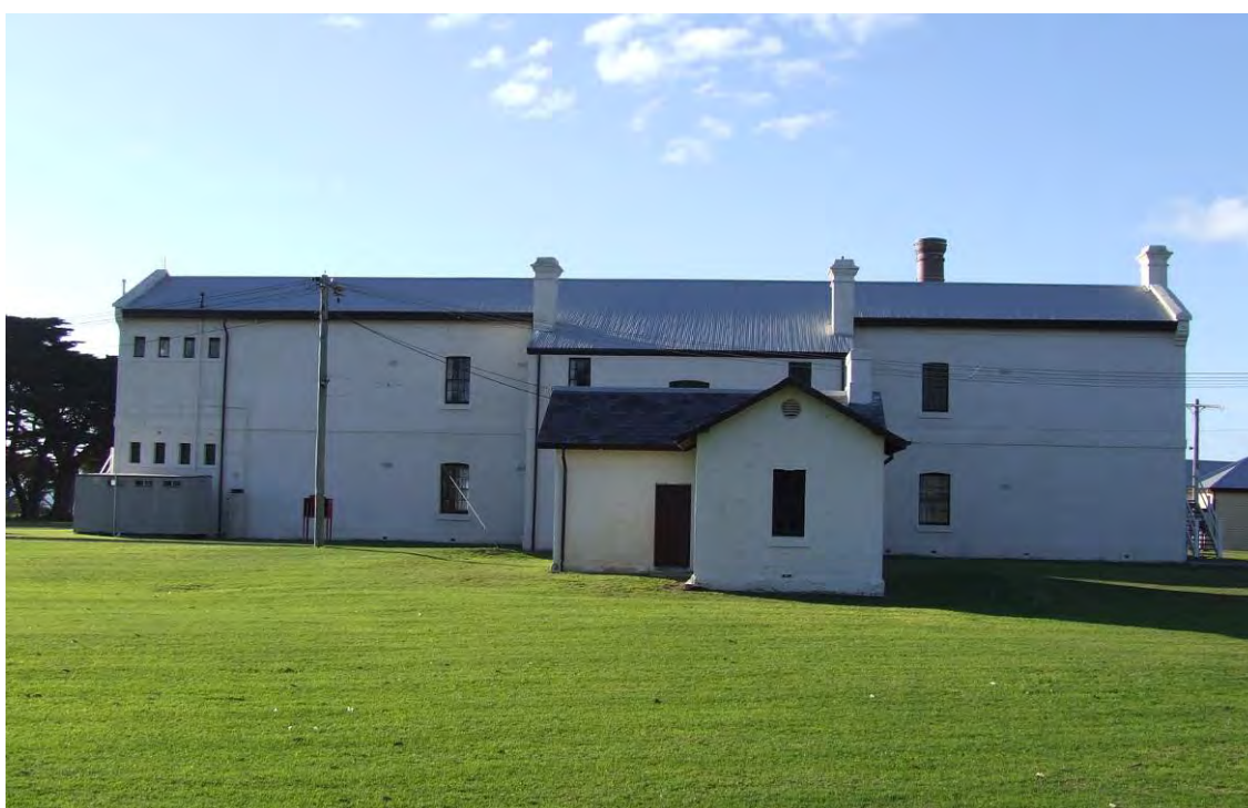
Figure 67 Image showing subject building in foreground, with Hospital No. 3 in background.
