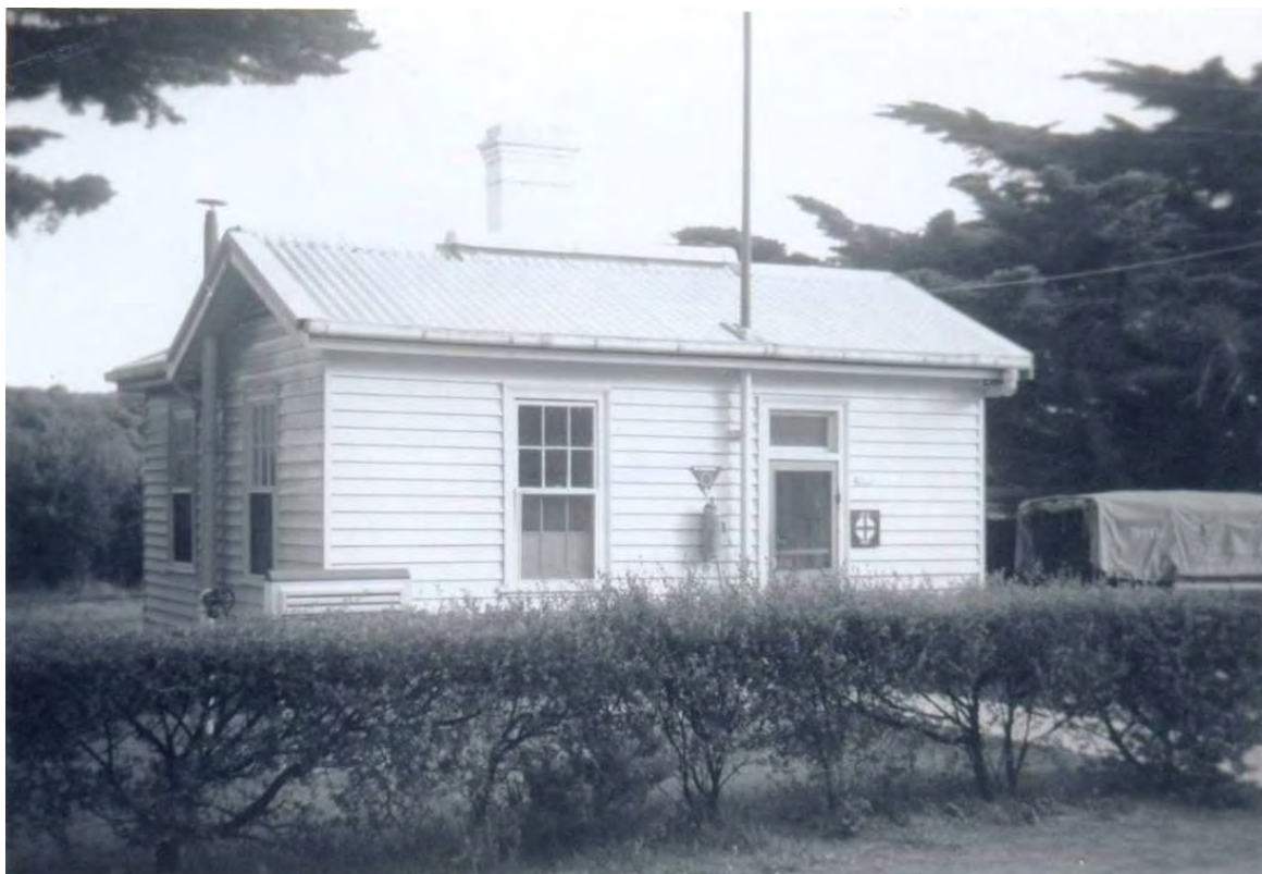
Figure 111 Building 26, photographed in May 1966.
