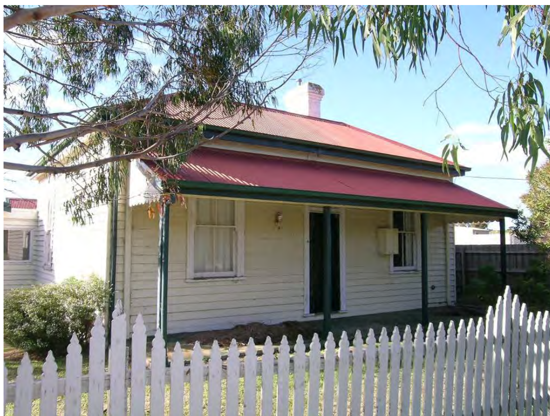
Figure 213 Building 1040, façade, facing south.
