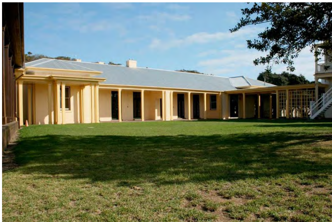
Figure 10 Building 3, north façade.
