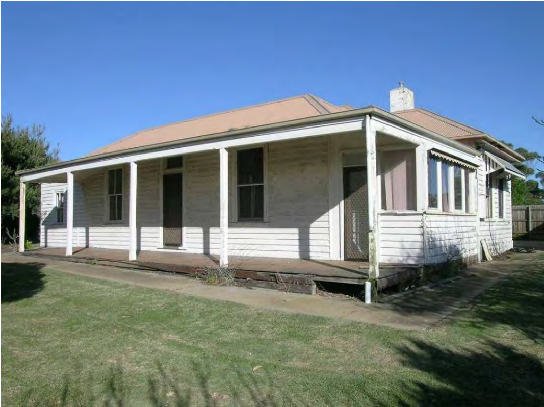
Figure 192 Building 966, showing the main north façade and part of the west elevation. Source: Courtesy Point Nepean Community Trust.
