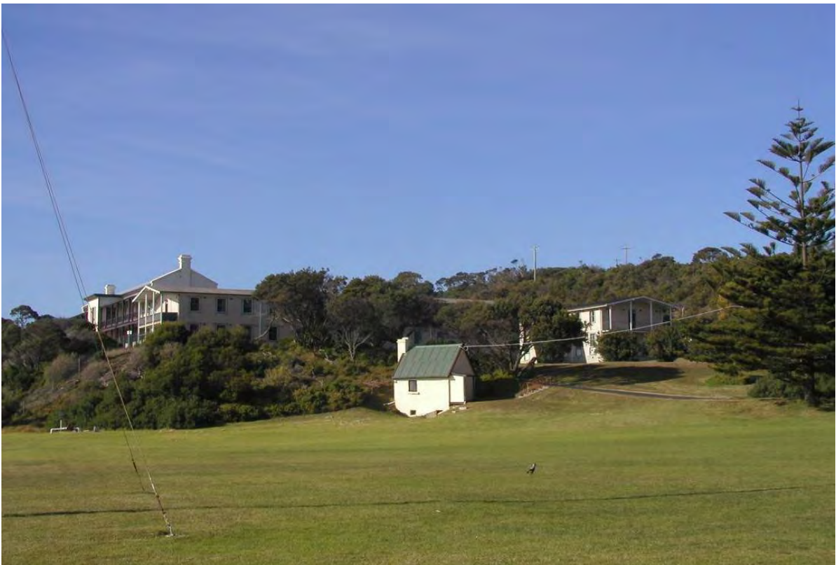
Figure 33 The subject building photographed in February 2008.
