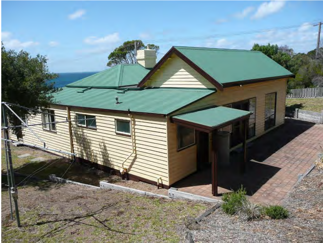
Figure 199 Building 1035, west and south elevations. The photograph clearly shows the phases of development, evident in the different roof forms.
