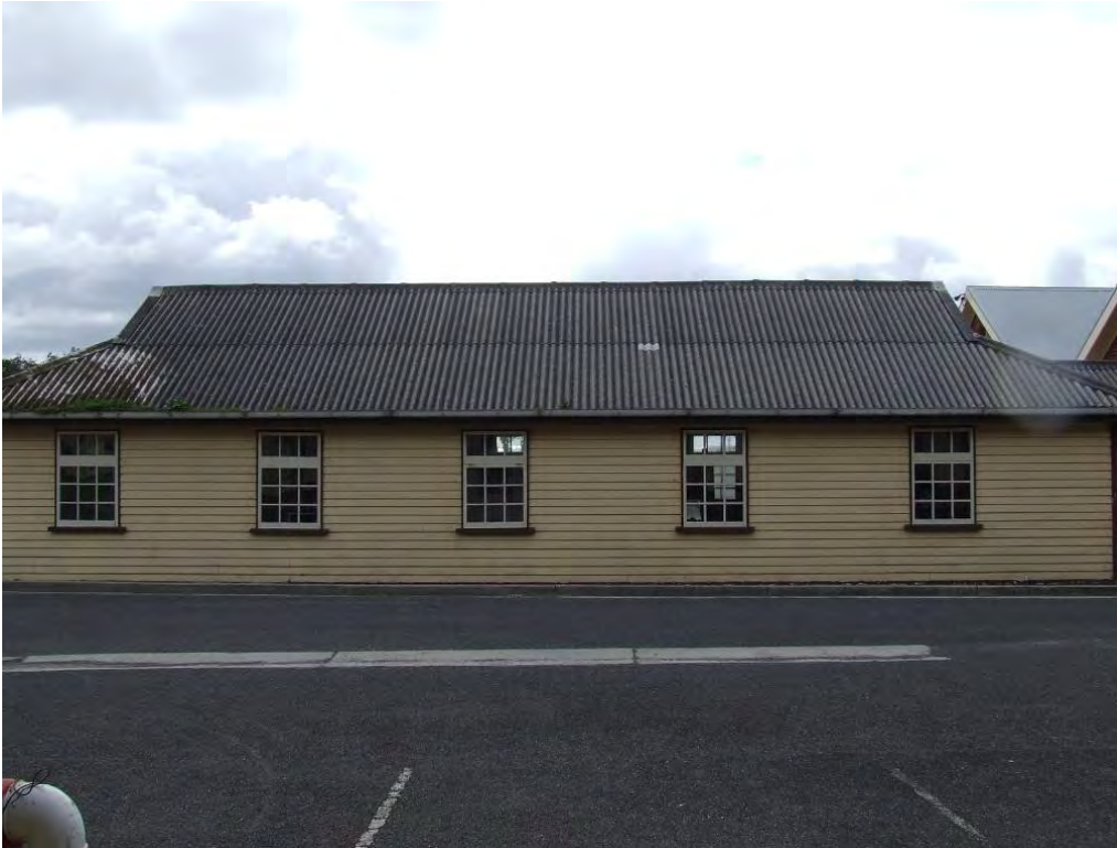
Figure 146 Building 62, south elevation.
