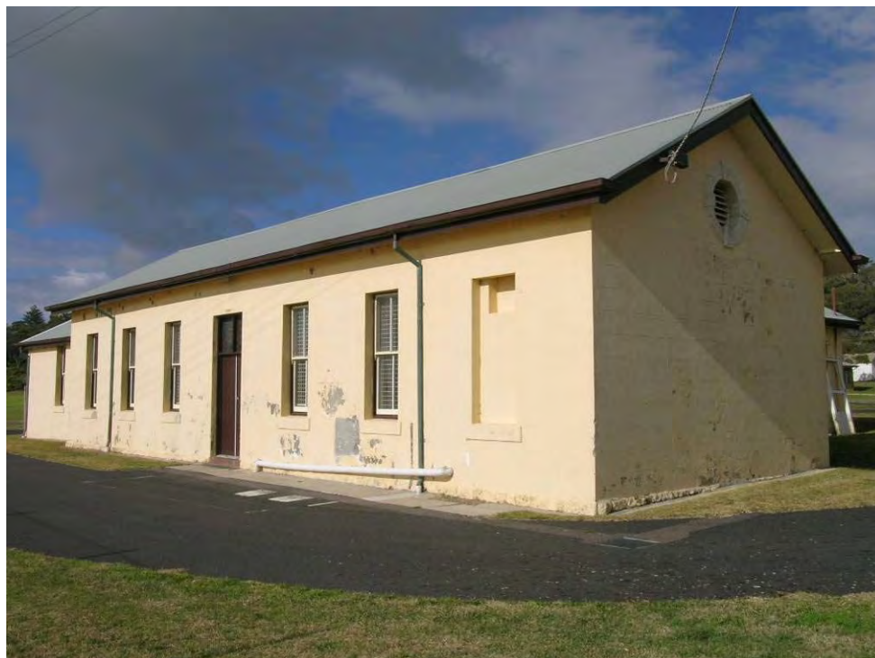
Figure 124 Building 59, showing the north and part west façades. The portion of the building to the far left is a subsequent addition.
