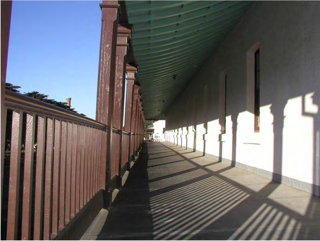
Figure 89 Building 22, looking east along the first floor verandah.
