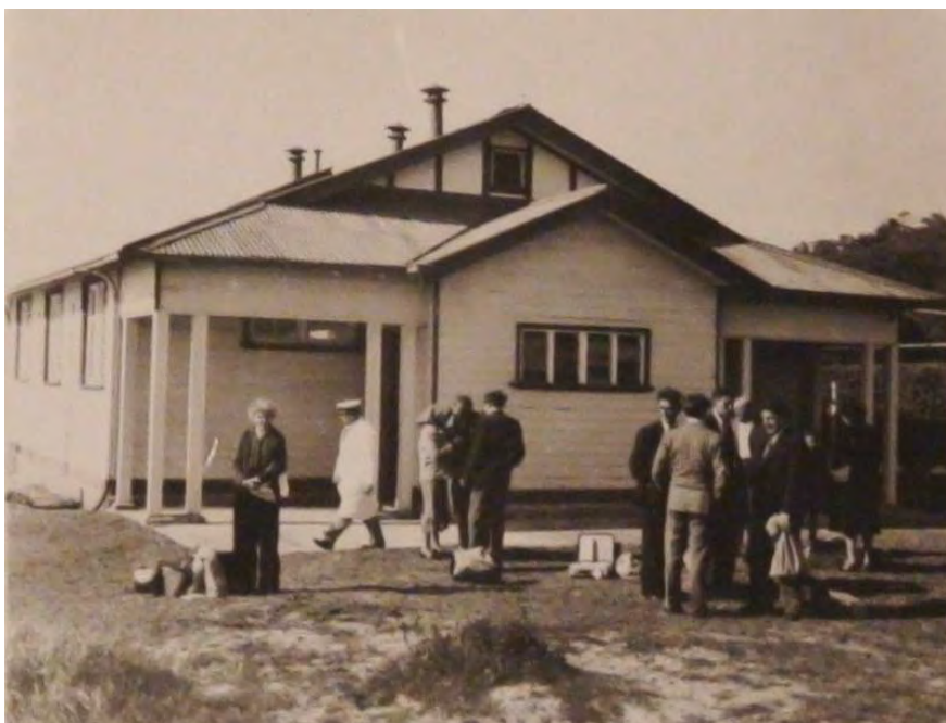
Figure 139 Undated photograph showing the west elevation of the shower block. Source: Fred Villiers collection, courtesy Point Nepean Community Trust.
