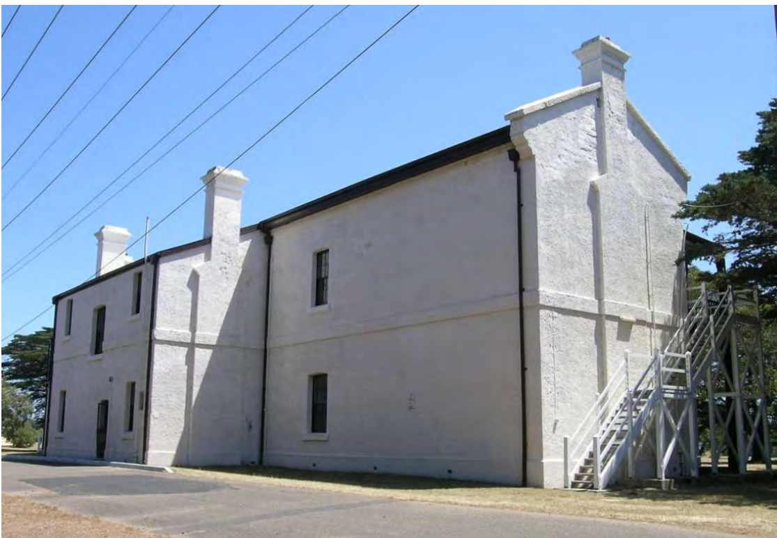
Figure 99 Building 25, southeast view from Bates Road.
