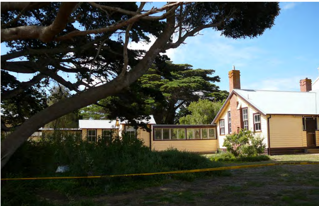
Figure 164 Building 65, showing its connection with Building 66. Note the covered way and the small servery – sited forward of the staff changing room. The covered way continued further west, connecting with Building 66. A high fence flanked the servery and changing room, dividing the administrative block from the hospital.
