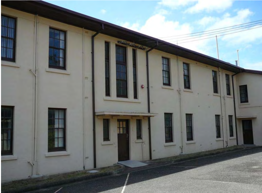
Figure 2 Building 1, partial view of south façade.
