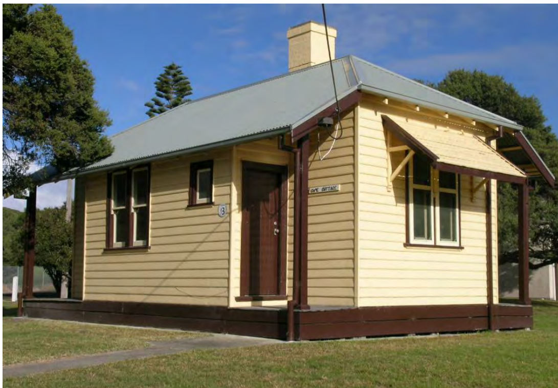
Figure 59 Building 13, northeast view.
