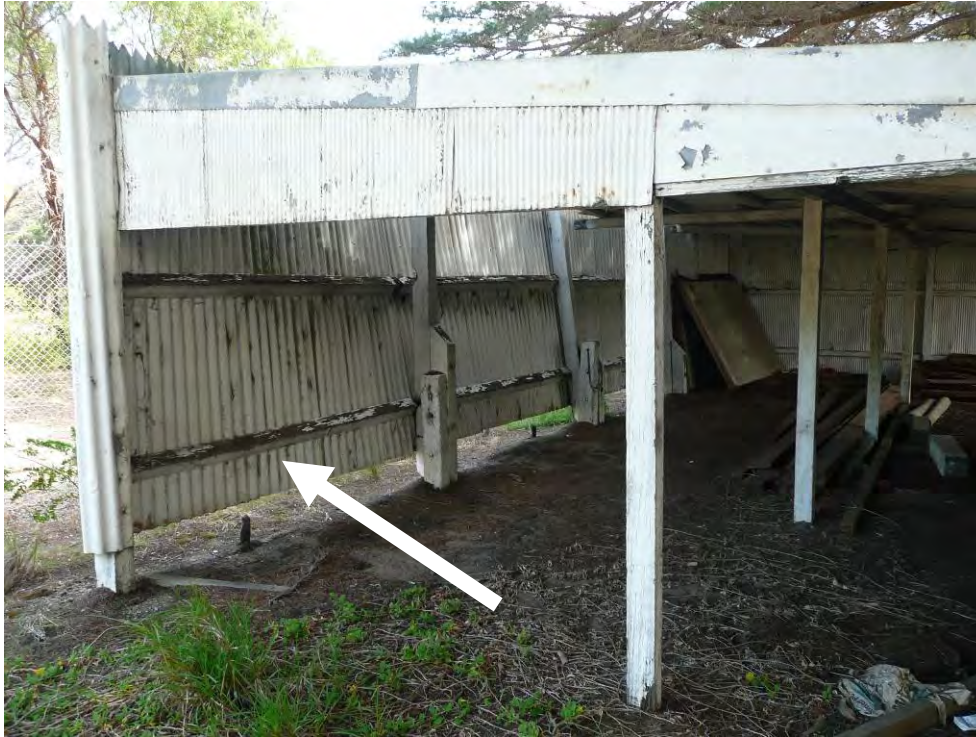
Figure 113 Building 27, showing the interior of the structure. The south elevation - indicated by the arrow - is thought to incorporate a portion of the original fencing to the Isolation Hospital compound.
