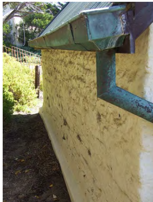
Figure 31 South façade and gutter detail
