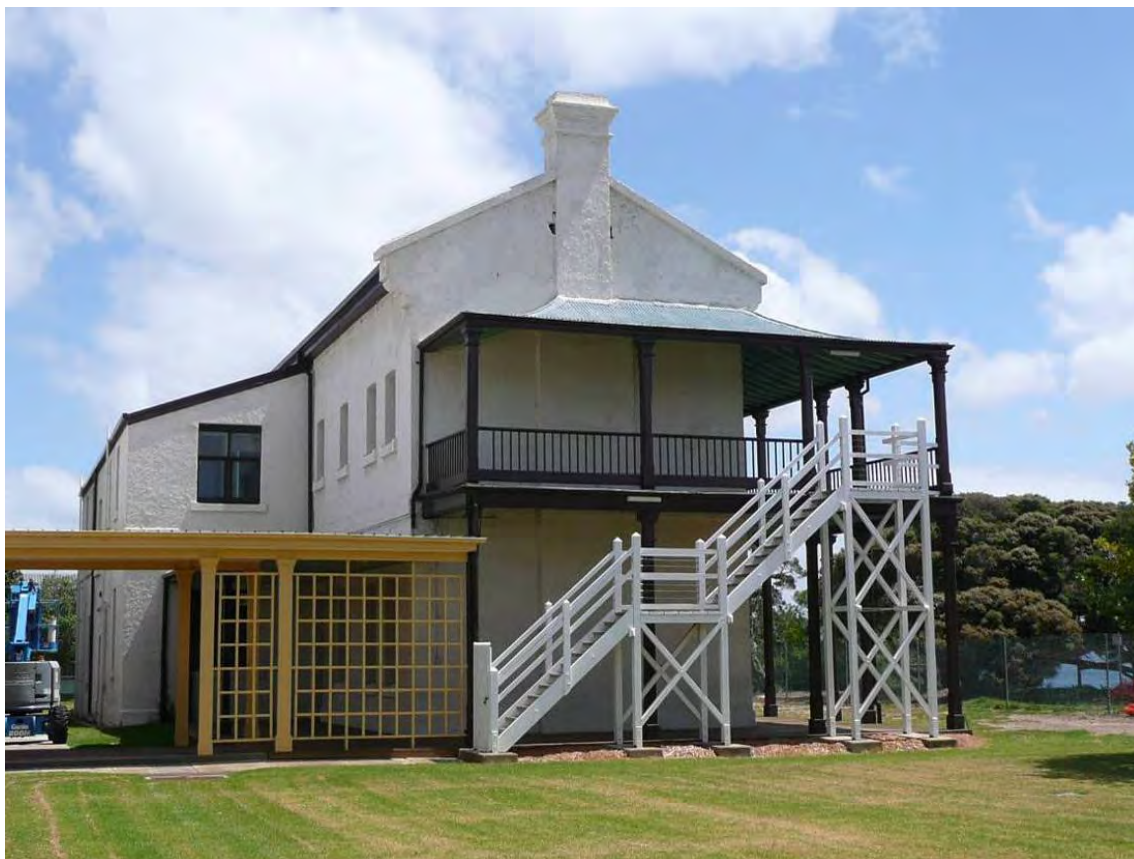
Figure 18 Building 4, southeast view.
