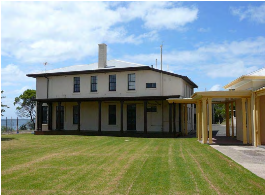
Figure 3 Building 1, west façade (the east façade is similar) – part of Building 3 can be seen at right.
