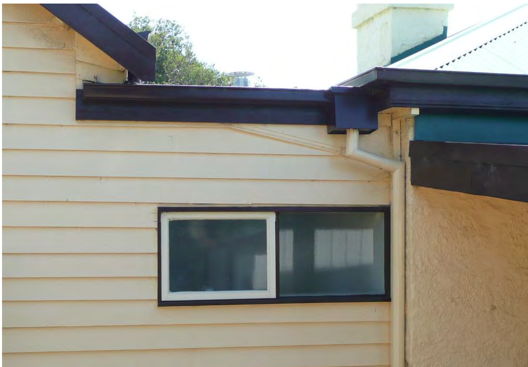
Figure 200 Building 1035, detail of the east elevation, showing the junction between the two phases of building with the verandah form of the timber addition expressed.
