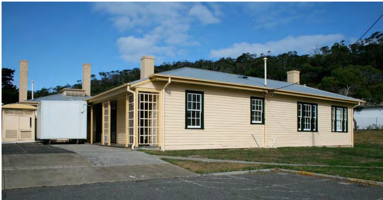
Figure 37 Building 9, northwest view. Note the early cool room structure to the extreme left of the image.
