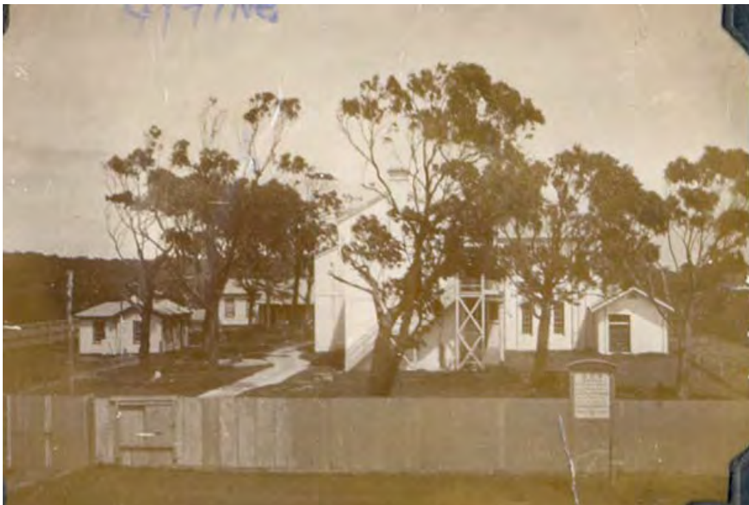
Figure 104 View of Building 25, from the same viewpoint, c.1920s, after the construction of the two-storey annexe (at right) and external stairs to building ends.
