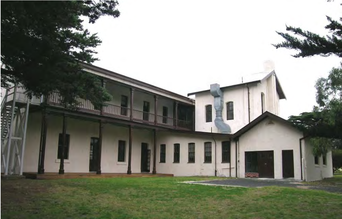
Figure 98 Building 25, northeast view.
