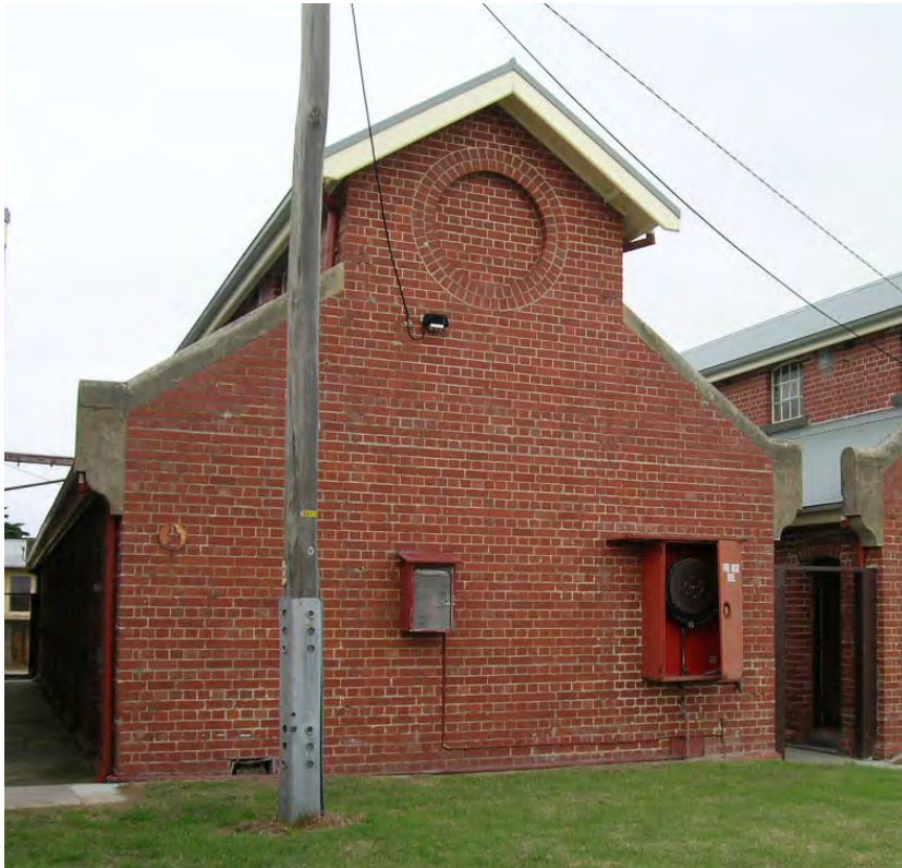
Figure 159 Building 64, detail of east elevation.
