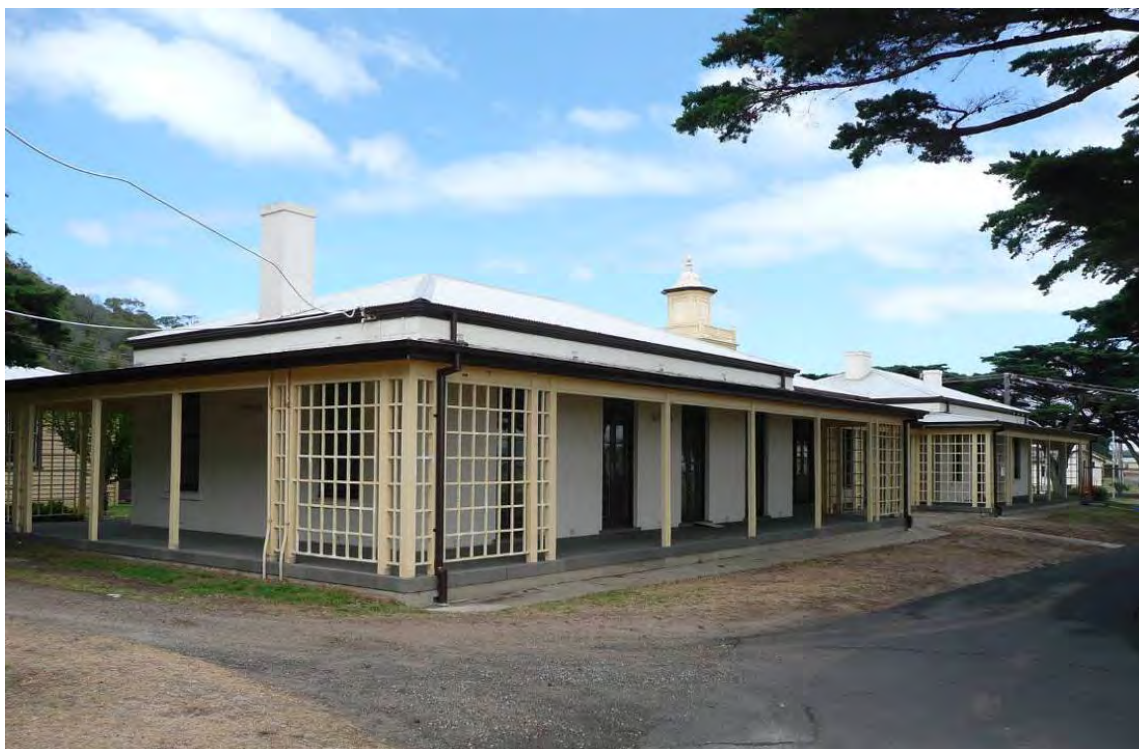
Figure 47 Building 10, showing part north and east facades.
