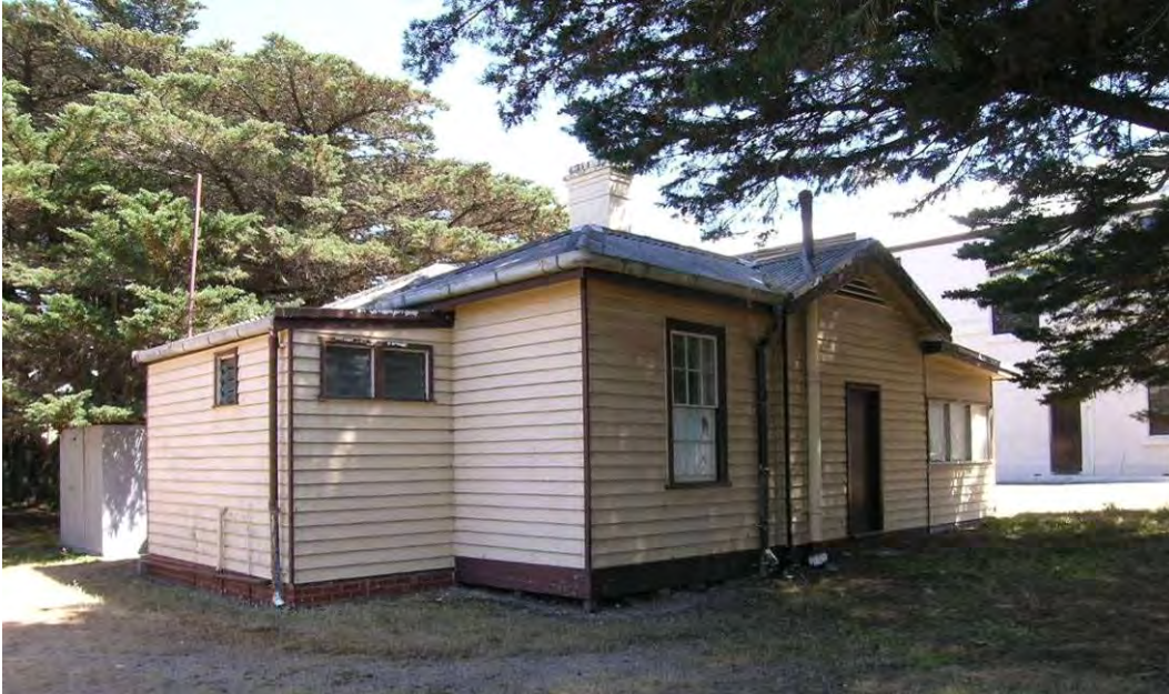
Figure 107 Building 26, showing the south and east elevations. Note the later skillion-roofed addition to the south elevation.
