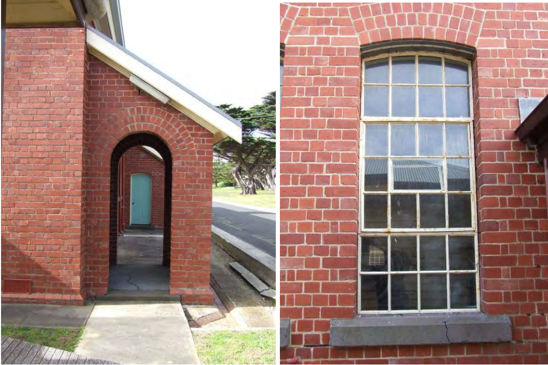
Figure 183 Building 84, from left: detail of brick semi-circular arch to west elevation; segmental arch window head over iron-framed multi-paned window to the east elevation.
