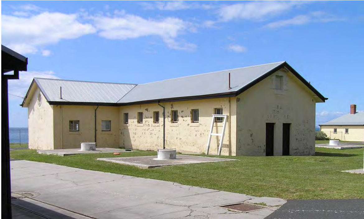
Figure 125 Building 59, looking north-east. Building 58 can be seen to the far right.
