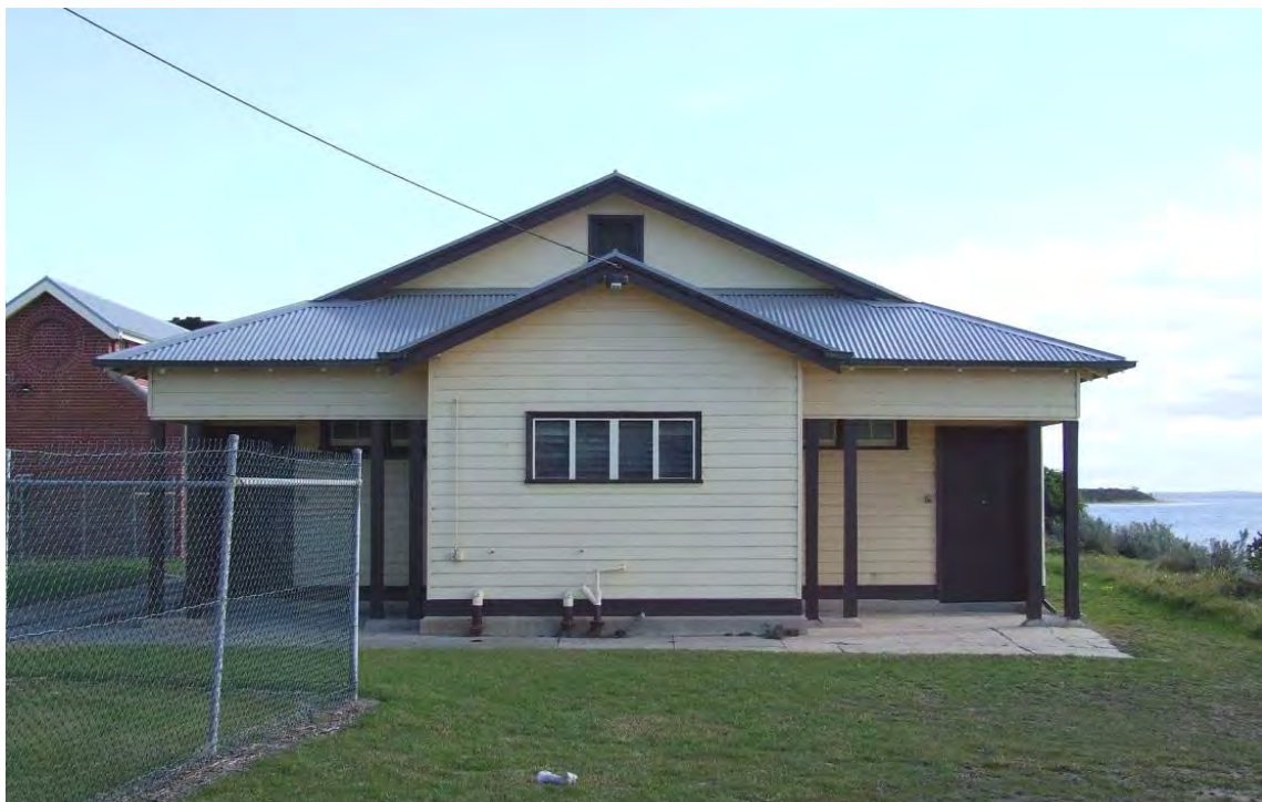
Figure 133 Building 60, showing the east (front) elevation. The toilet facilities are centrally located with flanking entrances to the segregated bathing facilities.
