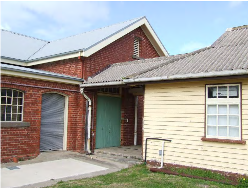
Figure 184 Building 84, west elevation showing the interconnection with Building 62, to where the clean luggage would be transferred by tram tray after the disinfection process.
