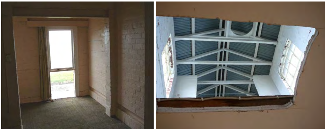
Figure 154 Building 63, from left: interior of one of the bathroom suites, later converted to accommodation; the lantern roof form above the bath chamber visible because of the removal of a section of the false ceiling.
