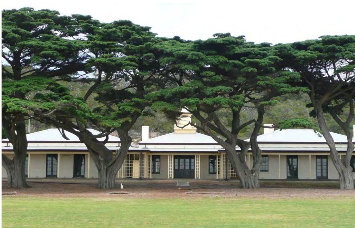
Figure 46 Building 10, viewed from the Parade Ground.
