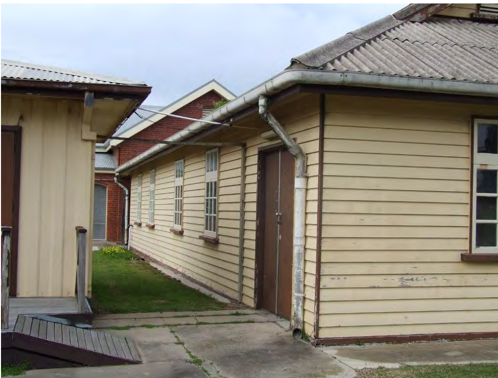
Figure 147 Building 62, north elevation and the inter-relationship with Building 84. Building 79 is at the left of the image.
