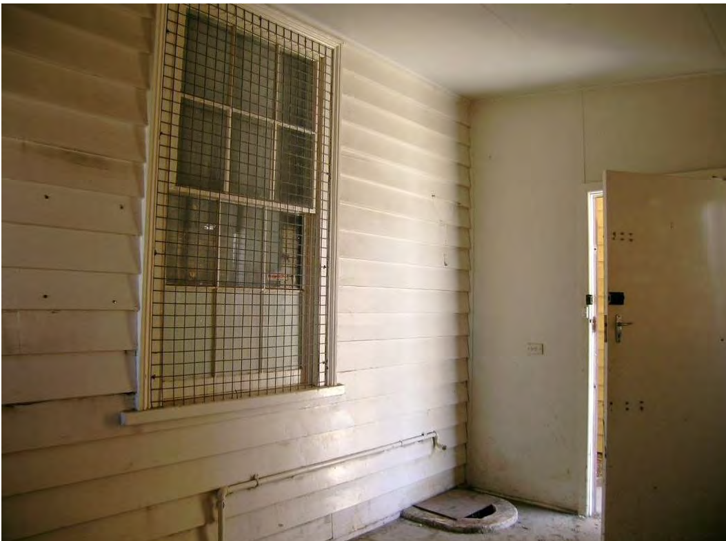
Figure 108 Building 26, showing the original façade now contained within the skillion-roofed addition. Compare with the photograph at Figure 111.
