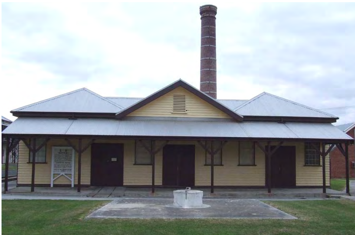
Figure 140 Building 61, showing the façade (east).
