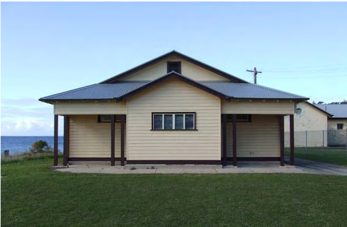
Figure 135 Building 60, showing the west (rear) elevation. The exit doors are located in the north and south walls of the central projecting bay.
