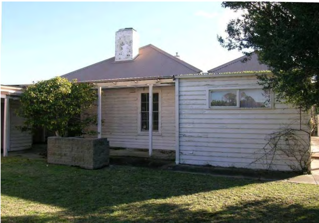
Figure 193 Building 966, showing the east elevation. Source: Courtesy Point Nepean Community Trust.
