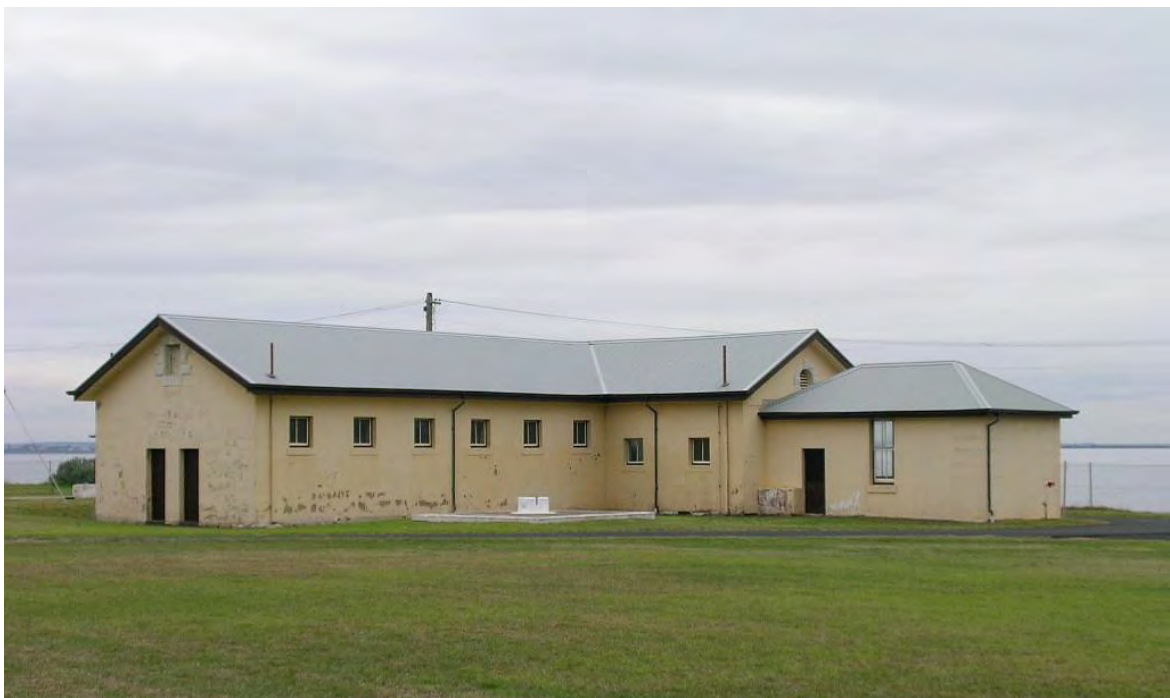
Figure 126 Building 59, looking north-west. The portion of the building to the far right (east side) is a later addition of the 1910s.
