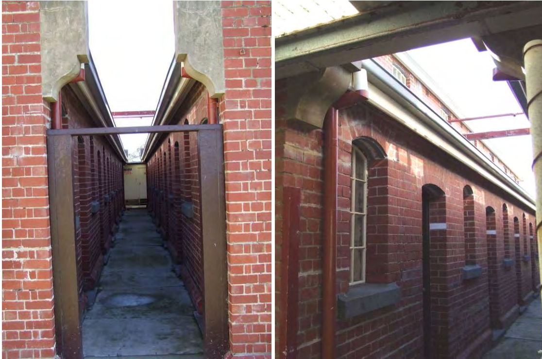
Figure 153 Buildings 63 and 64, from left: looking west down the central access way or 'alley' between the two bath houses; the steel-framed window forms and doorway detailing of Building 63. Note the recent repairs and strengthening works to the segmental brick window heads.
