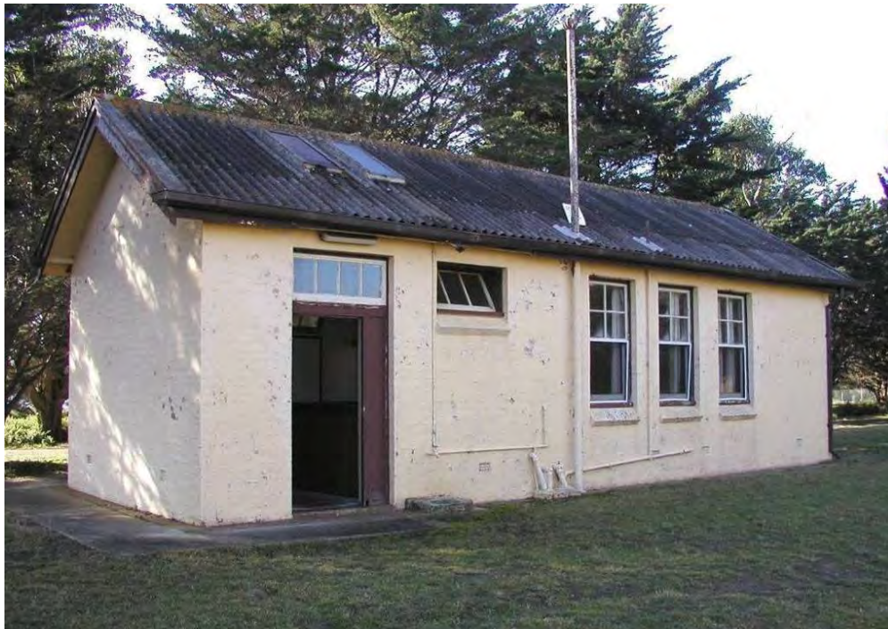
Figure 176 Building 67, south elevation. The open door leads into the former mortuary room.
