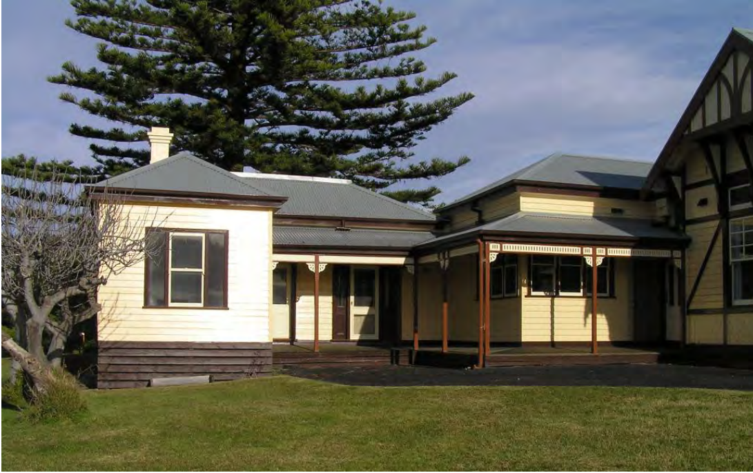
Figure 205 Building 71, north elevation and part of Building 1038.
