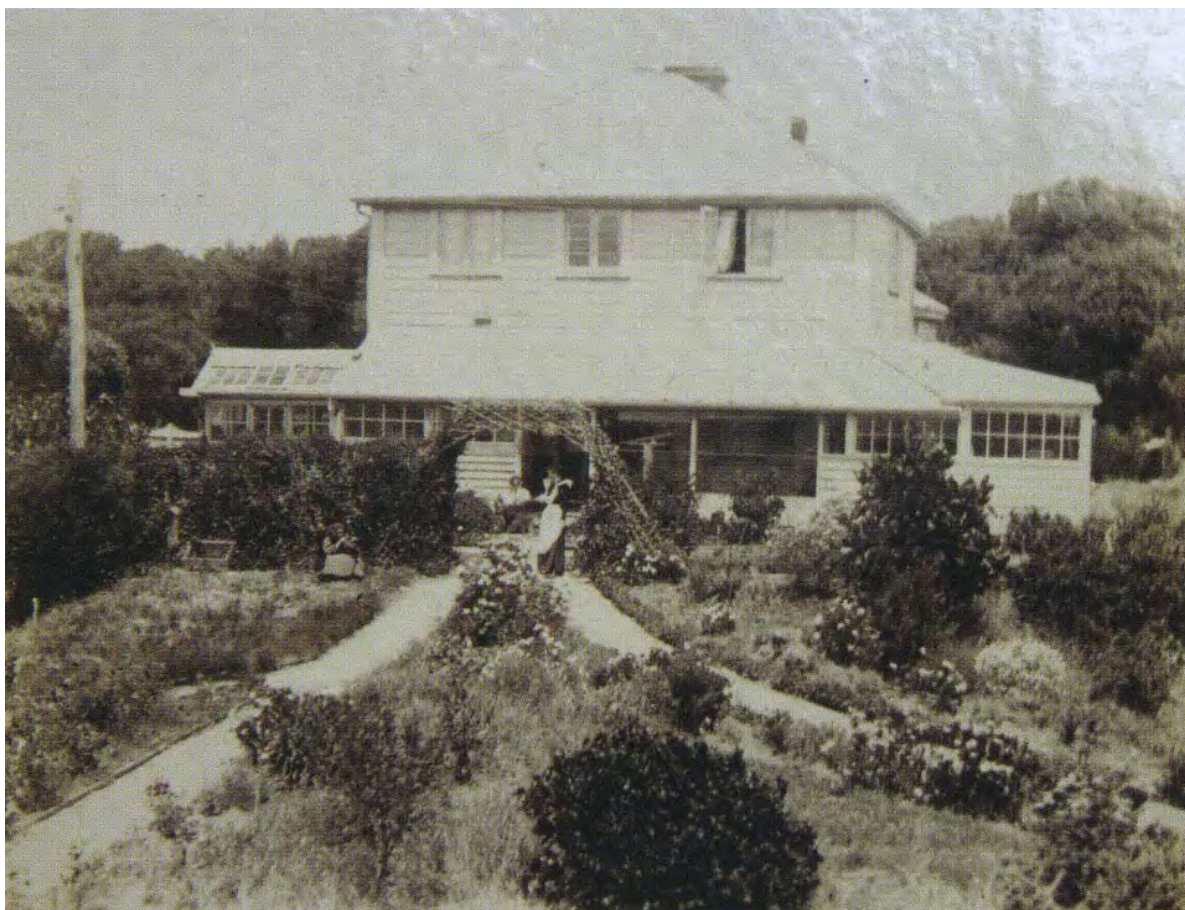
Figure 207 View from the north – the photograph is thought to date from somewhere between 1885 and c.1899 Source: Nepean Historical Society.
