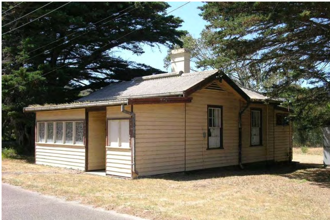
Figure 106 Building 26, showing the north and west elevations, from Bates Road. Note the later skillion roofed addition to the façade.
