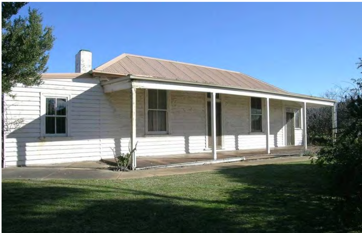
Figure 191 Building 966, façade, facing northeast.
