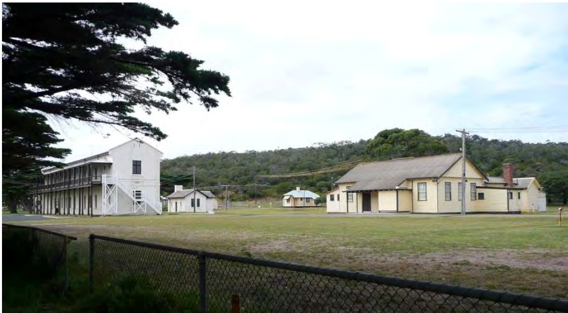
Figure 78 View looking south-east showing north-west facades of Building 18. Other buildings are Building 16 (far left), Building 15 (left of centre), and Building 13 (centre).
