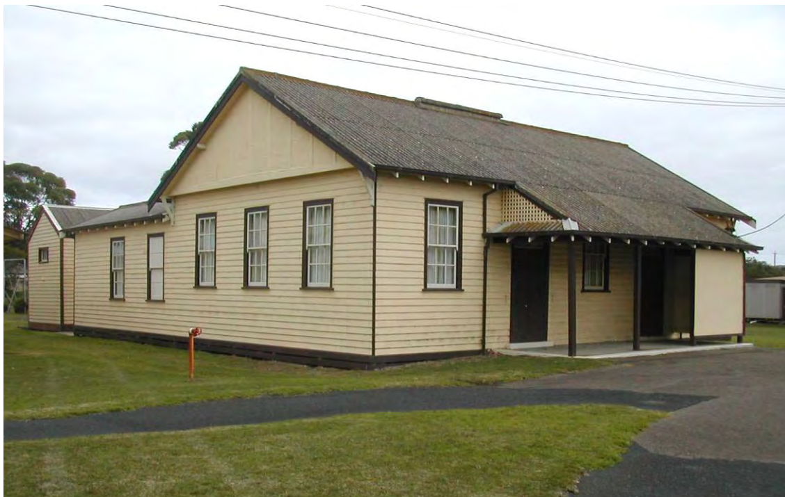
Figure 76 Building 18, showing the east and north façades. Building 19 is partly visible to the rear.
