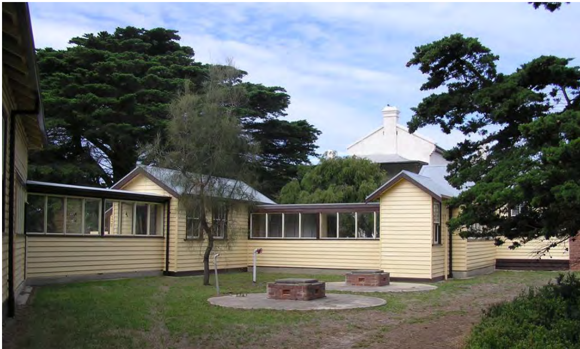
Figure 172 Building 66, looking east towards Building 65. The gable west end of Building 25 (Hospital No. 5) is in the background. The staff changing room and servery are the two interlinked structures. Note the two capped wells in the centre of the image.
