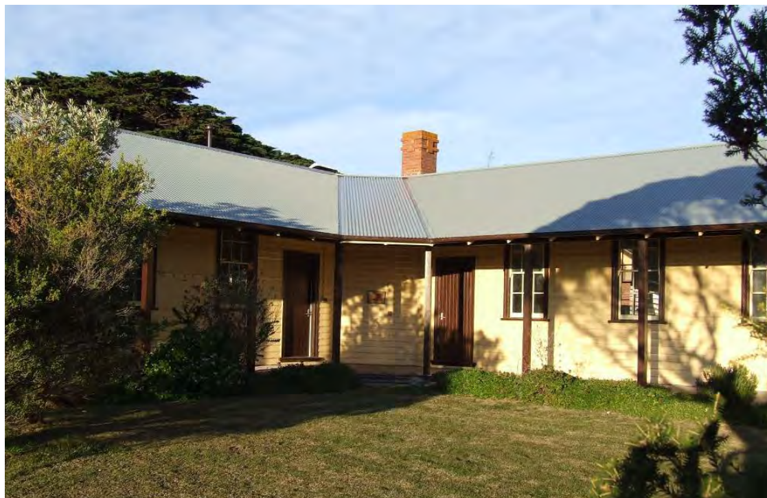
Figure 170 Building 66, looking east and showing the central garden area between the two ward blocks/wings. At the centre of the image is the wall of the Duty Room.
