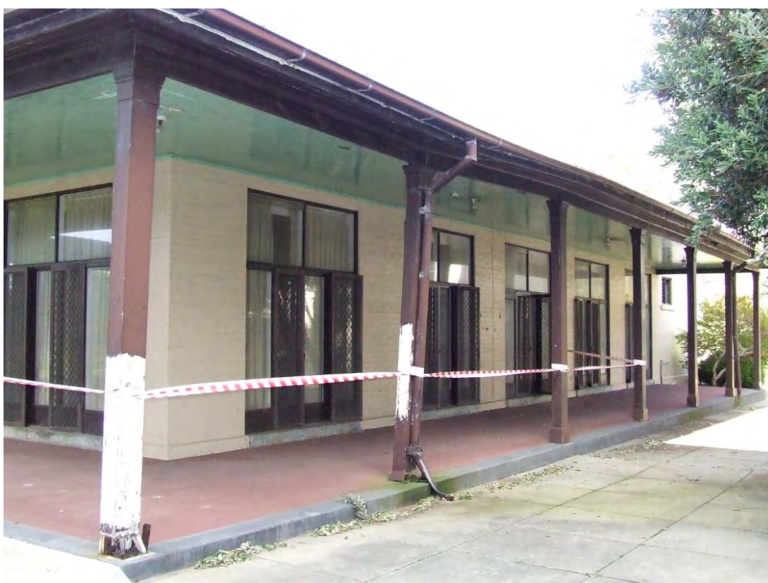
Figure 12 Building 3, showing the mid-1960s west extension. The photograph shows the building prior to the programme of recently completed restoration works.
