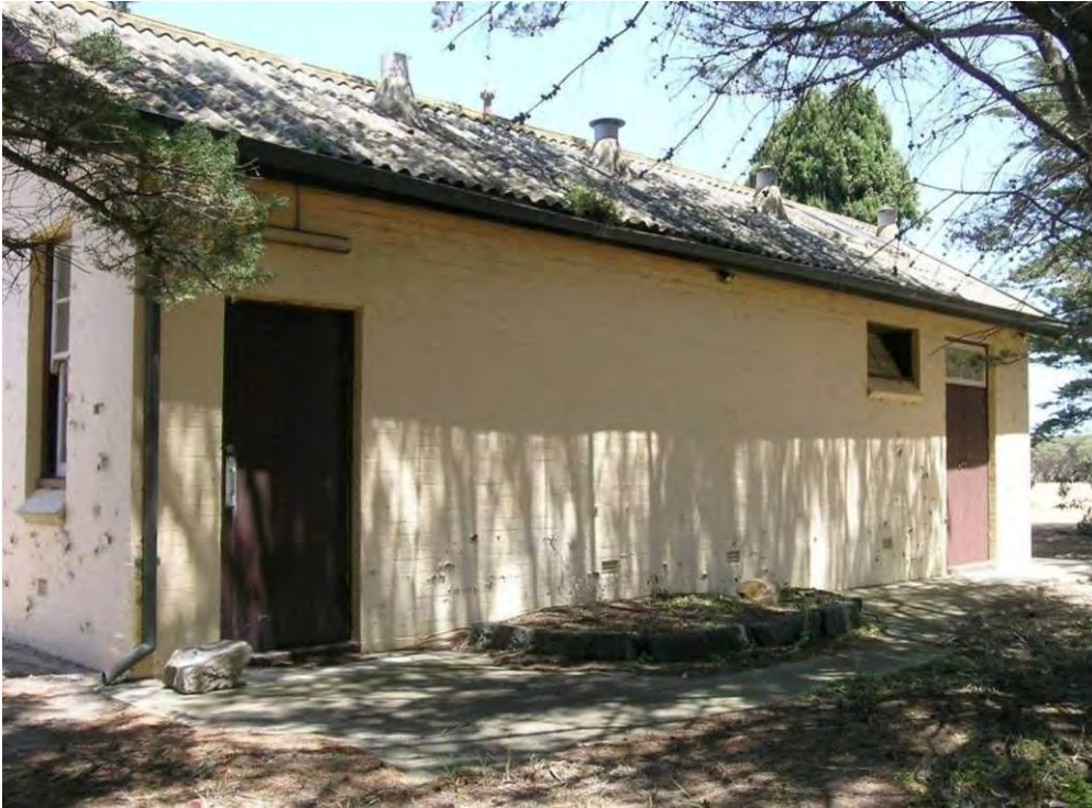
Figure 177 Building 67, north elevation. The door at left provides access to a small lobby to the former laboratory and the door at right provides access to the former mortuary room.
