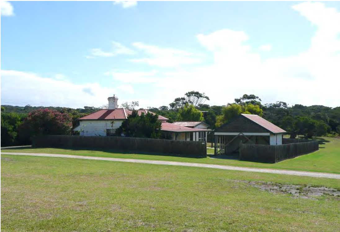
Figure 215 Building 1040, showing the east and north elevations from the adjacent Police Point Reserve.
