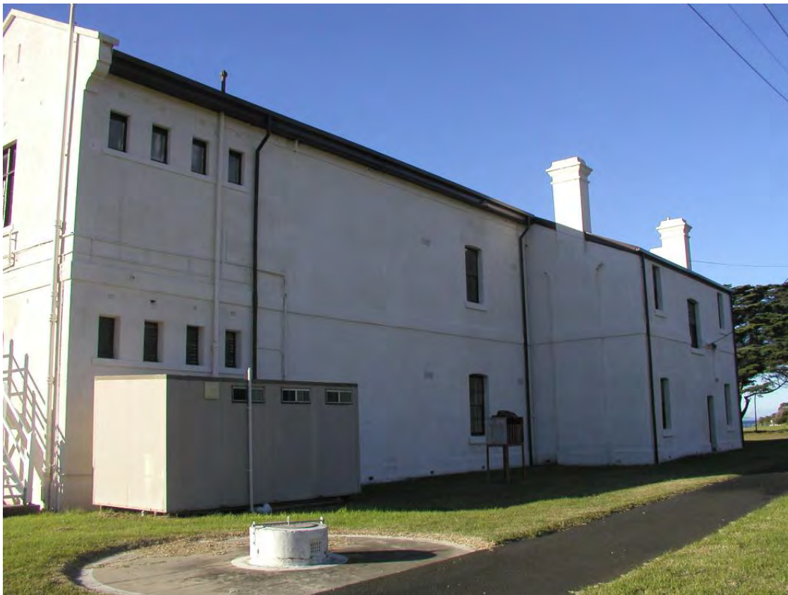
Figure 71 Building 16, showing the south façade – the c.1916 addition to the west end of the original hospital building is clearly identified by the rows of small windows on the left of the image.
