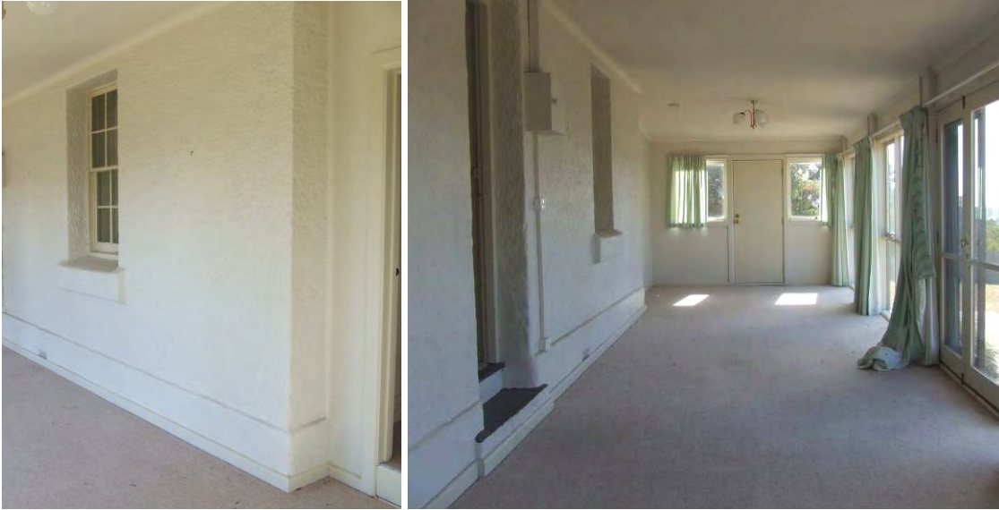
Figure 201 Building 1035, from left: original window of the 1857-58 cottage, now enclosed within the verandah; the enclosed verandah looking west. The original front door opening is at left.
