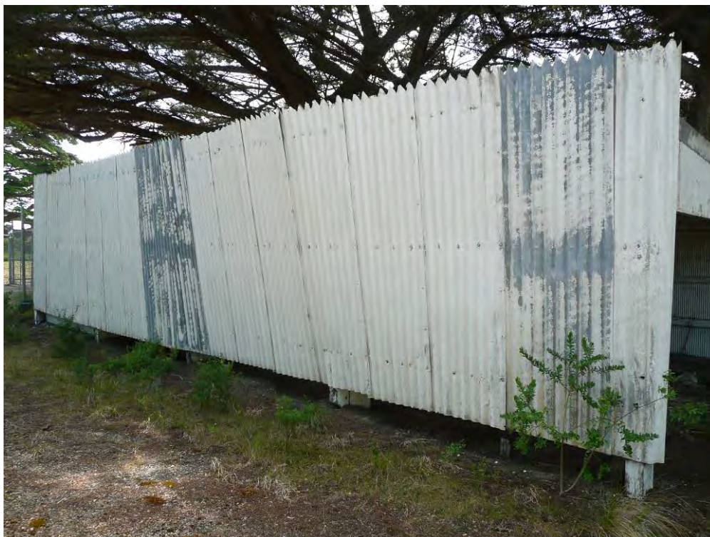
Figure 112 Building 27, showing the south elevation of the structure.
