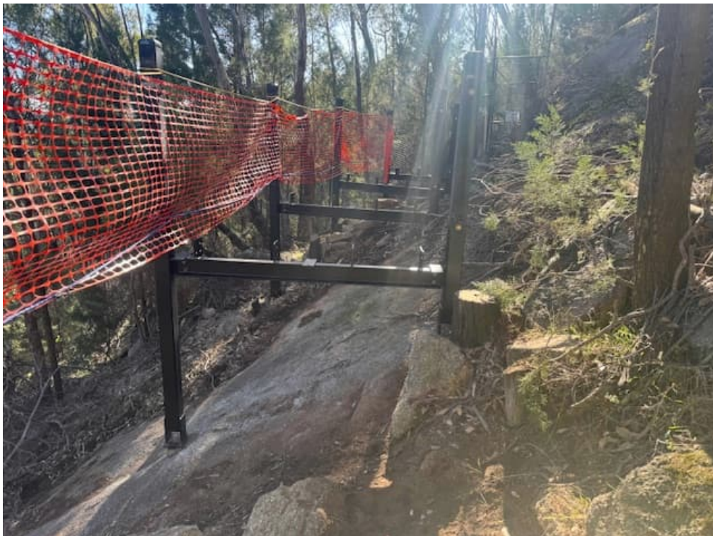
Photo 24 Topcoat Painting complete (up to FSL)
