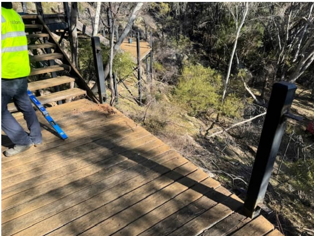
Photo 12 Balustrade removal
