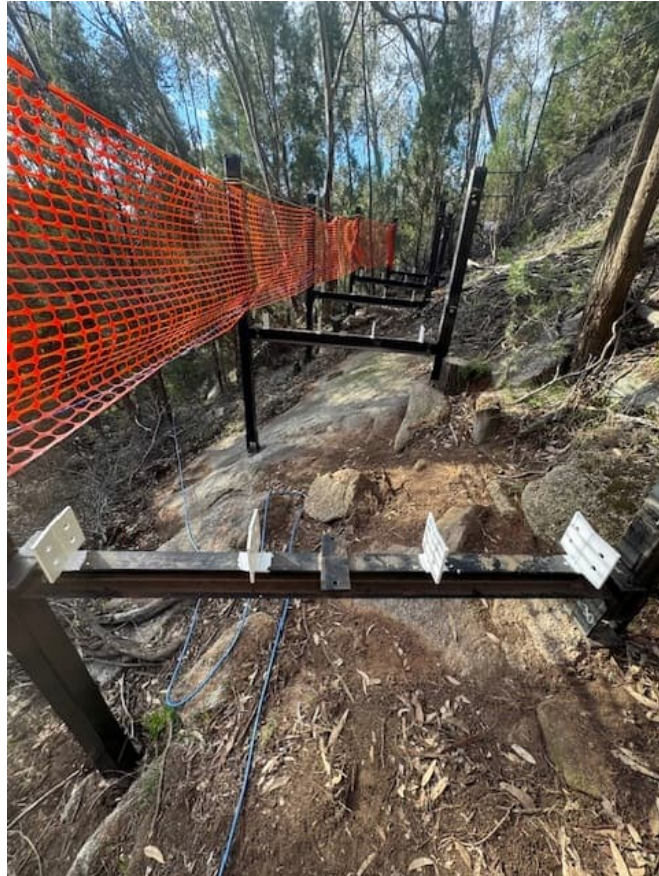
Photo 19 Cleat epoxy paint – 2 x coats
