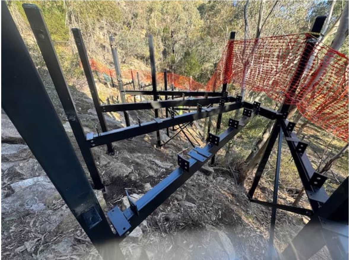
Photo 25 Topcoat Painting complete (up to FSL)
