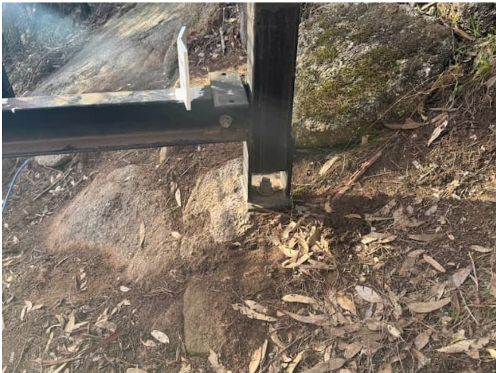
Photo 20 Base of posts exposed
