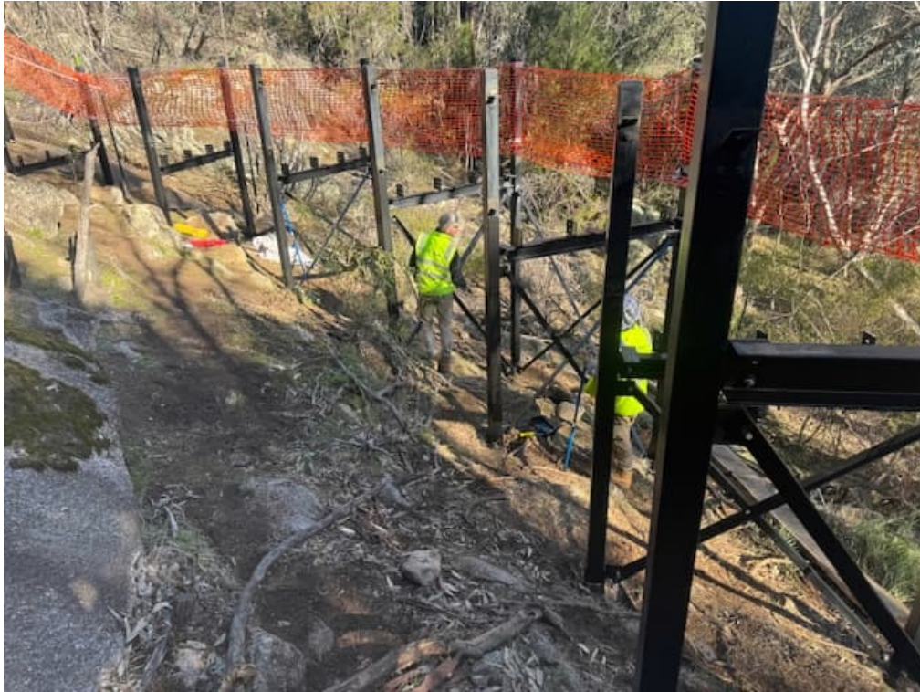
Photo 23 Topcoat Painting complete (up to FSL)
