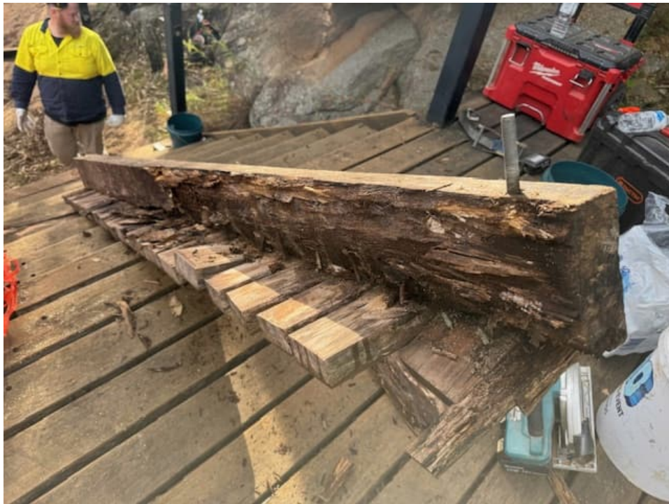
Photo 15 Existing Joist removal
