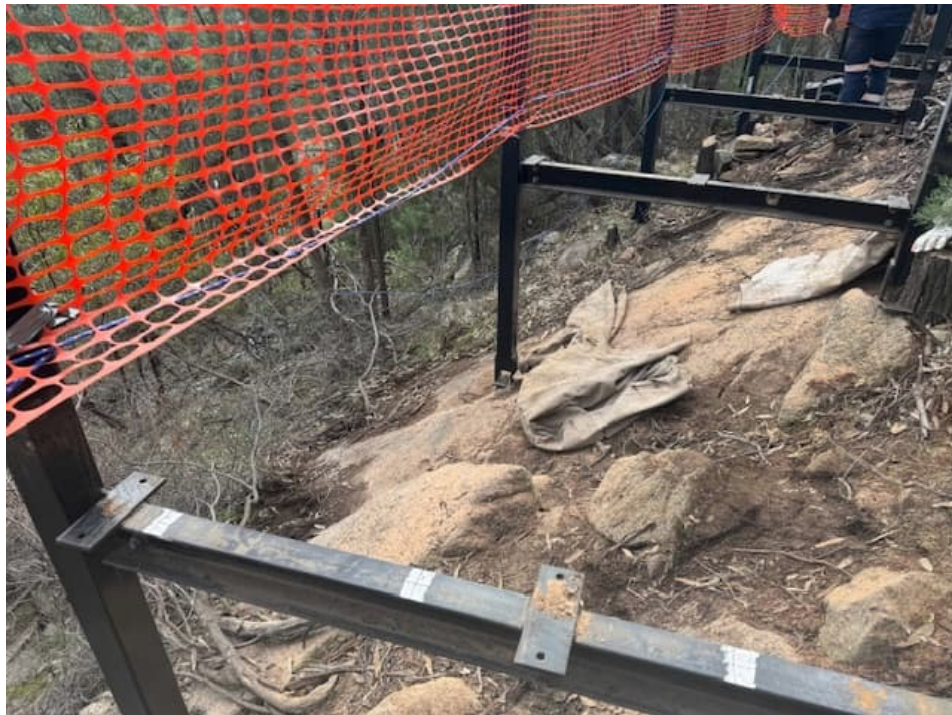
Photo 17 Joist cleat surface prep
