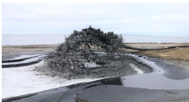
Dredged sand is transferred through pipes to the disposal site
