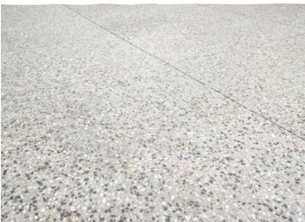
**Figure 55: Potential Activity Node Pavement:** *Coloured Concrete Pavement with Lightly Exposed Aggregate*
