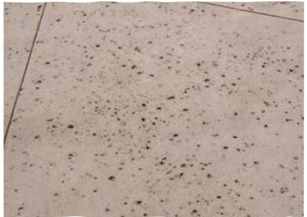
**Figure 57: Potential Activity Node Pavement:** *Coloured Concrete Pavement with Salt Finish*
