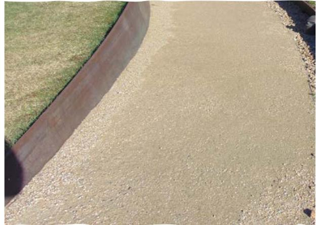
**Figure 56: Shared Path Pavement:** *Granitic Gravel with Cement Stabiliser*
