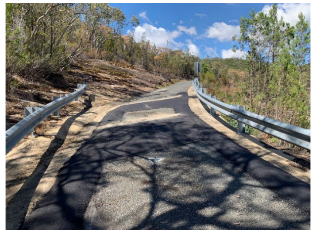
Above: Raised bitumen sections were installed to direct water away from the bridge. New stone drains help water run off the road.
