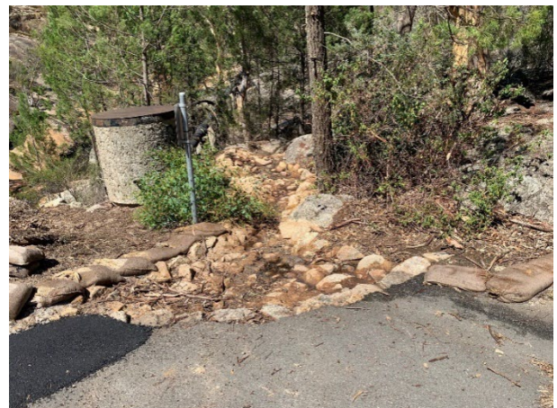
Above: new stone drains help protect the bridge from stormwater damage.
