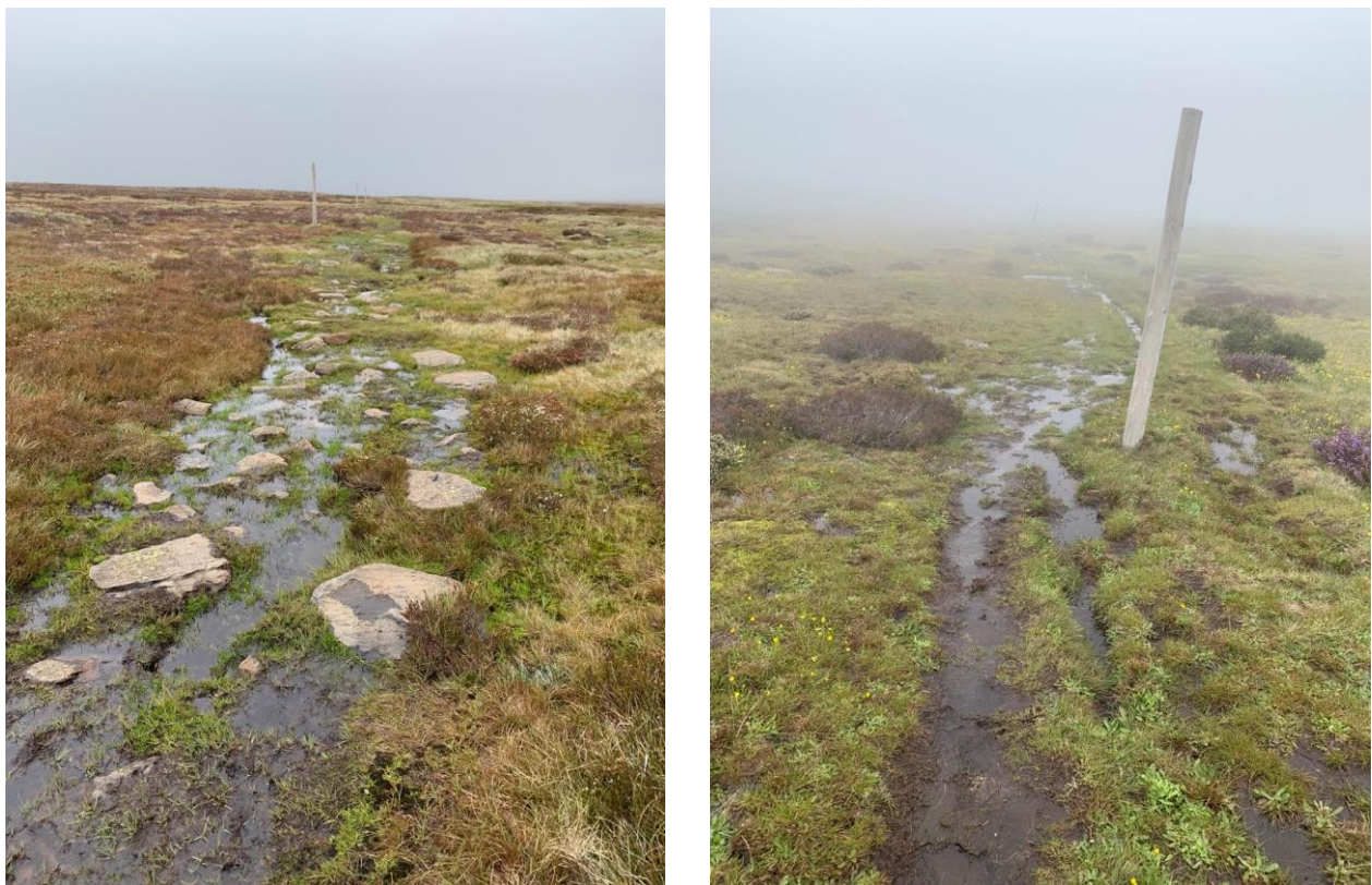
Figure 9 Examples of sections of trail with poor drainage (credit Parks Victoria)
