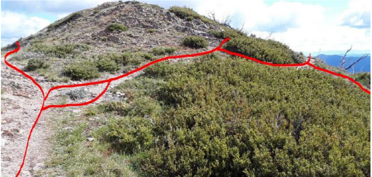
Figure 8 Example of poorly defined track impacted by branching (credit Abzeco)
