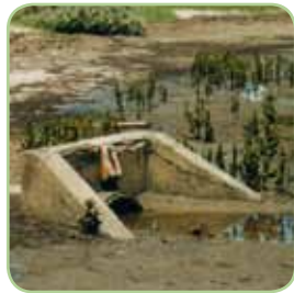
▲ Drains discharging stormwater in a concentrated flow can upset the salinity balance, scour mudflats, cause erosion and deposit high nutrient loads.
