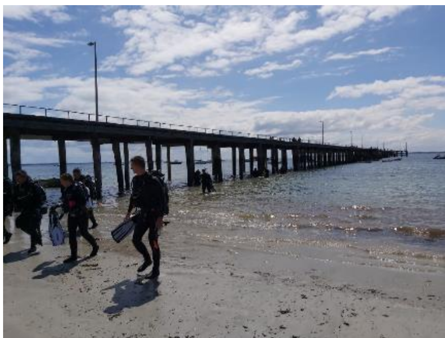
Figure 6. SCUBA diving school emerge after dive at Flinders Pier
