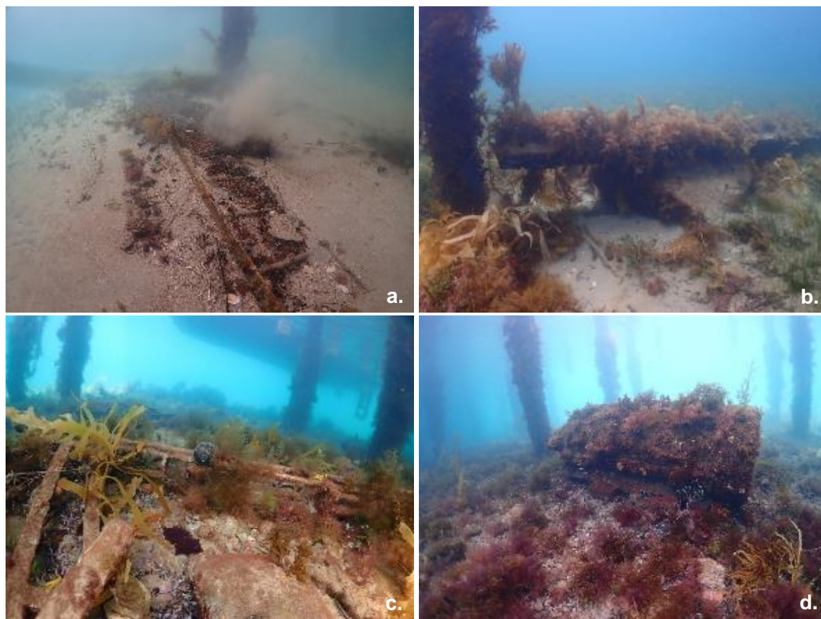
Figure 34. Debris under the Flinders Pier, December 2020.
