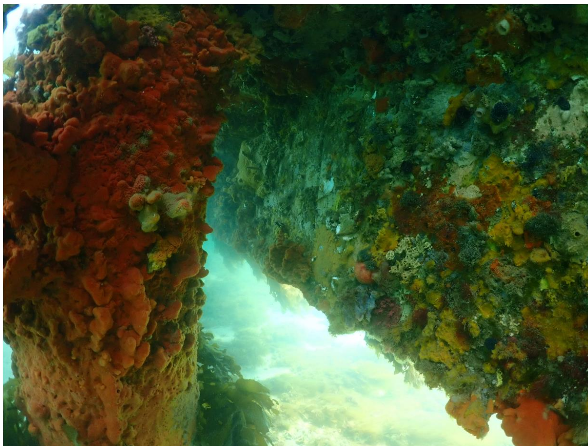
Figure 68. Outer steel pile and concrete wave screen at Blairgowrie, 2021
