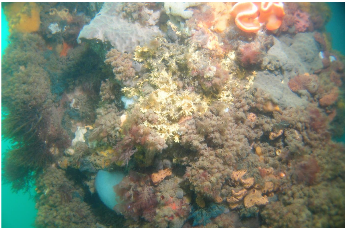
Figure 69. Encrusting invertebrates on steel jetty pile, North Arm Western Port
