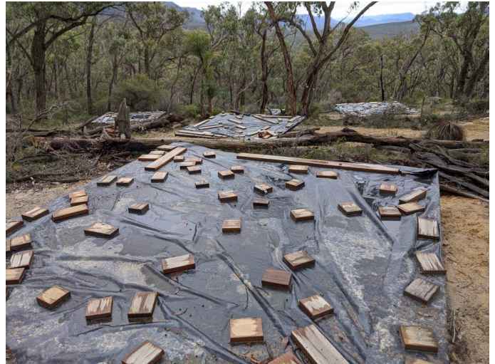
Above: Construction of tent pads at Djardji-Djawara (Cassidy Gap).
