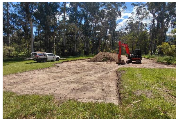
Earthworks have begun for the new carpark and entry point.
