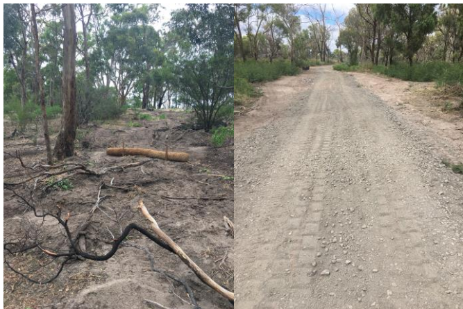
Trail rehabilitation works
