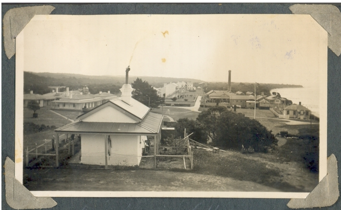
Figure 13 c.1920s/30s view of the Quarantine Station clearly showing the stone surgery in the foreground. Source: Devereux-Gray album, courtesy Point Nepean Community Trust.
