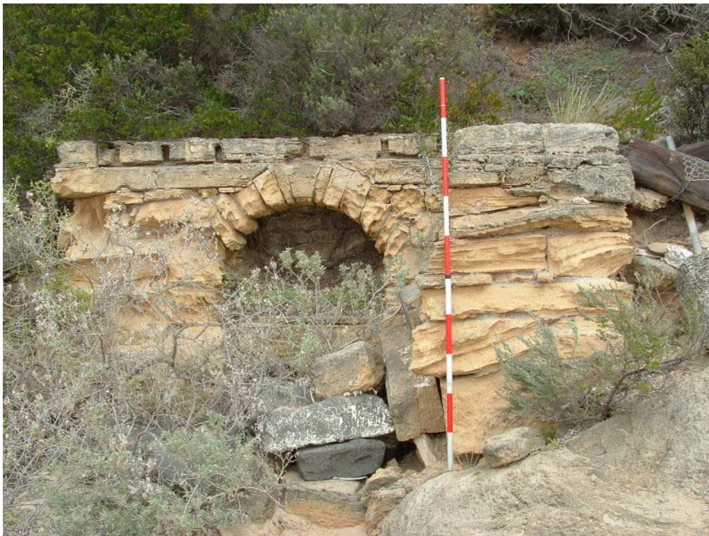
Figure 71 Image of Lime Kiln 2.
