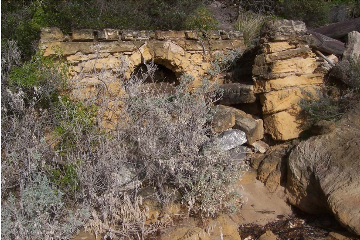
Figure 72 Another view of Lime Kiln 2.
