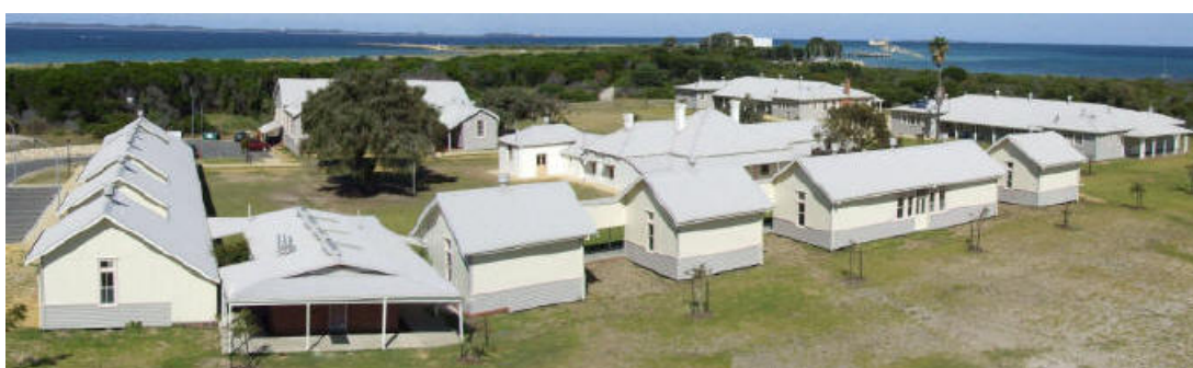
Figure 74 Buildings at the Woodman Point Quarantine Station, at Munster, WA. The accommodation buildings are single storeyed and the buildings at the extreme left were built as Ships Crew quarters.
