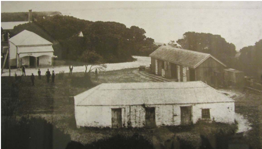
Figure 8 View of early station buildings, c. 1890. In the foreground is Patrick Sullivan's stone house, requisitioned in response to the Ticonderoga landing of 1852 and behind – to the left – is the stone store, one of the first buildings erected, using emigrant labour in 1853. The building to the rear right is a timber stables. These buildings (long demolished) are on the site of the current Parade Ground. Source: Courtesy Point Nepean Quarantine Station Museum.
