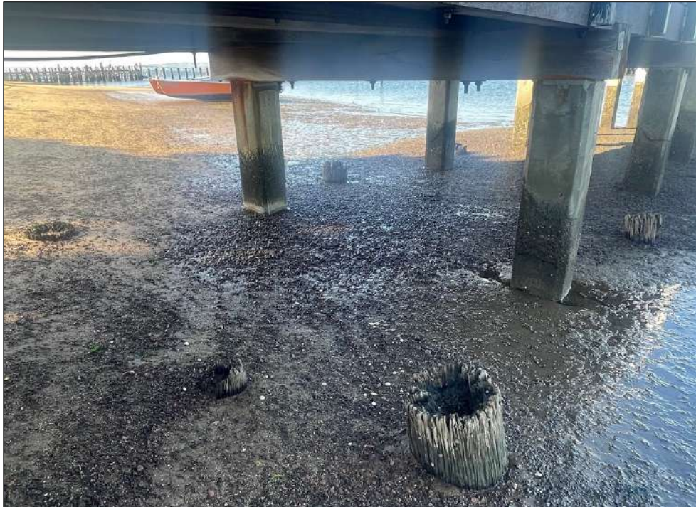
Figure 26 Remnants of earlier timber piles below the jetty. Note the current piles are concrete.
