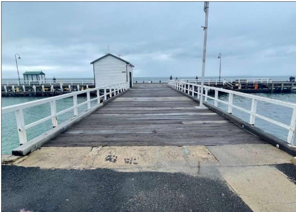
Figure 30 View of the pier where it transitions from the stone mole to the timber T-head.
