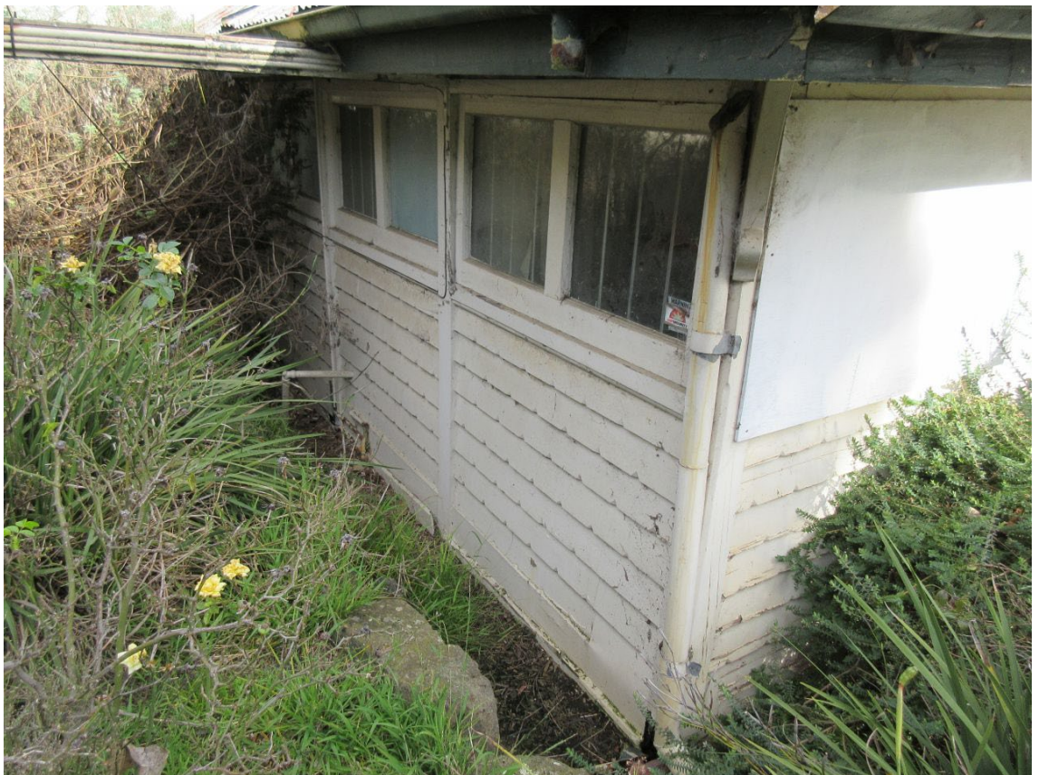
Figure 54 The rear elevation of the Curator's Office
