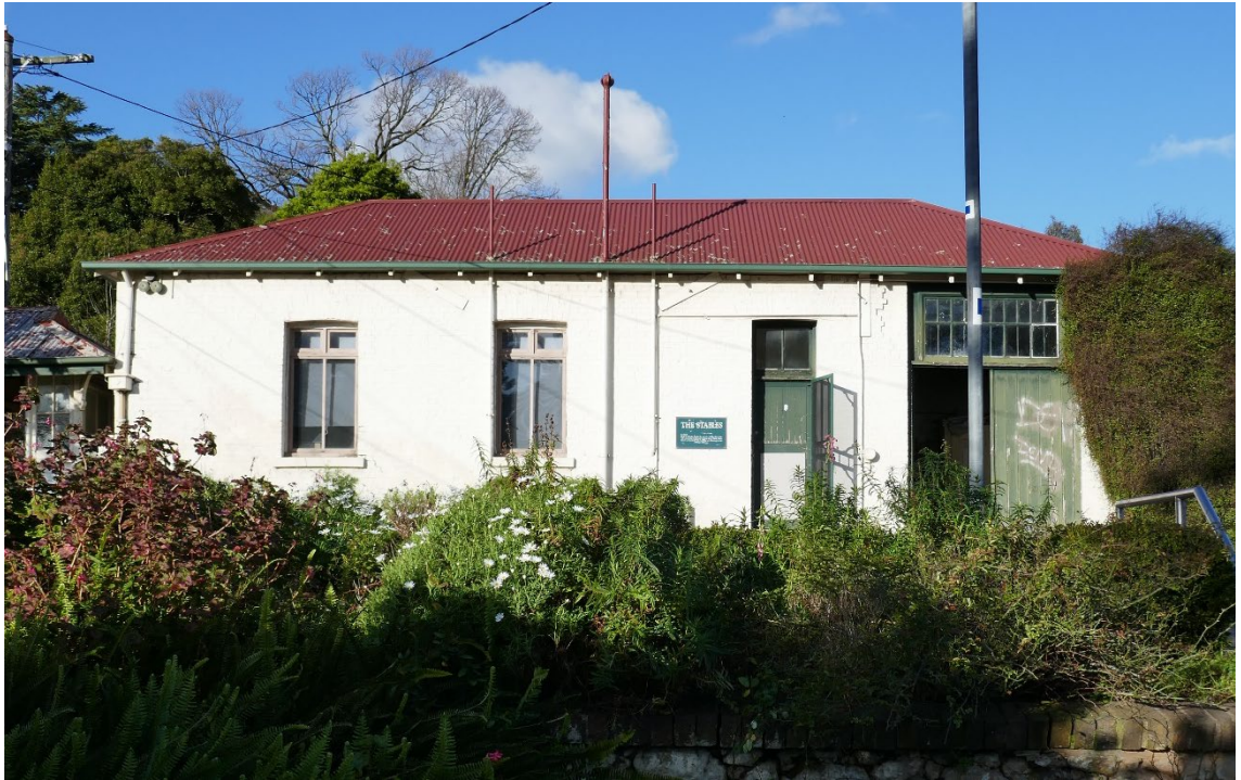
Figure 29 Front (east) elevation of the Stables
