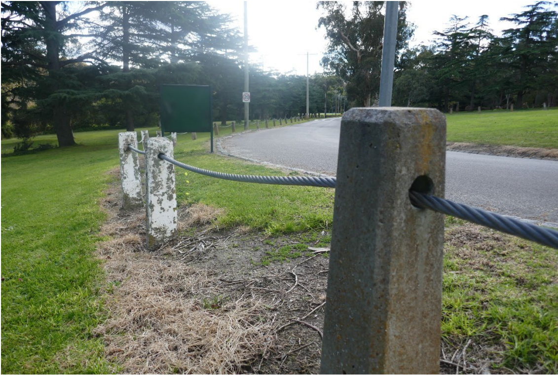
Figure 58 The age, condition and presentation of the concrete bollards varies
