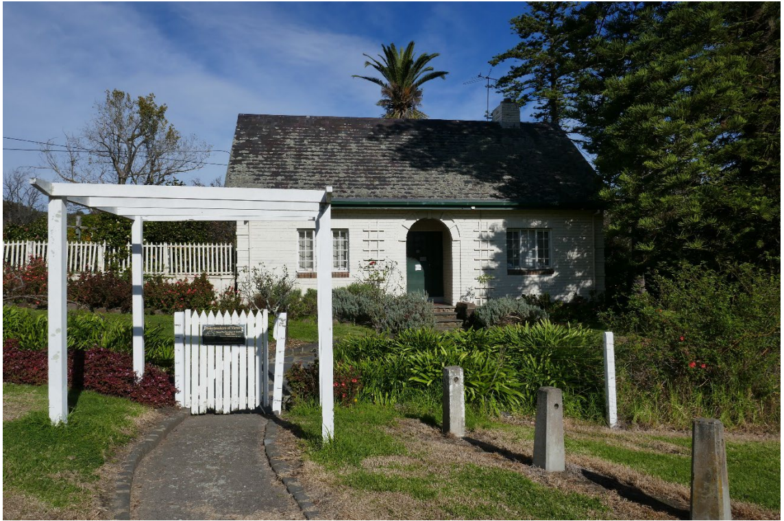
Figure 27 Front (north) elevation of the curator's cottage
