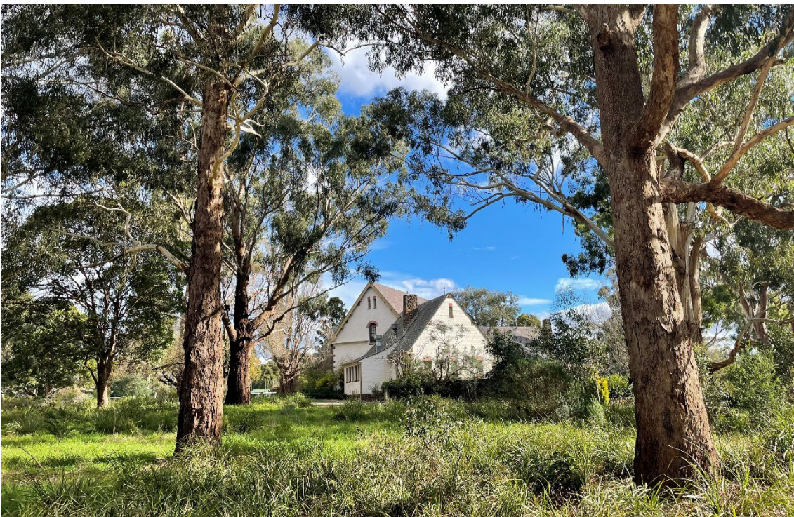
Figure 16 View of the Chalet from the picnic area
