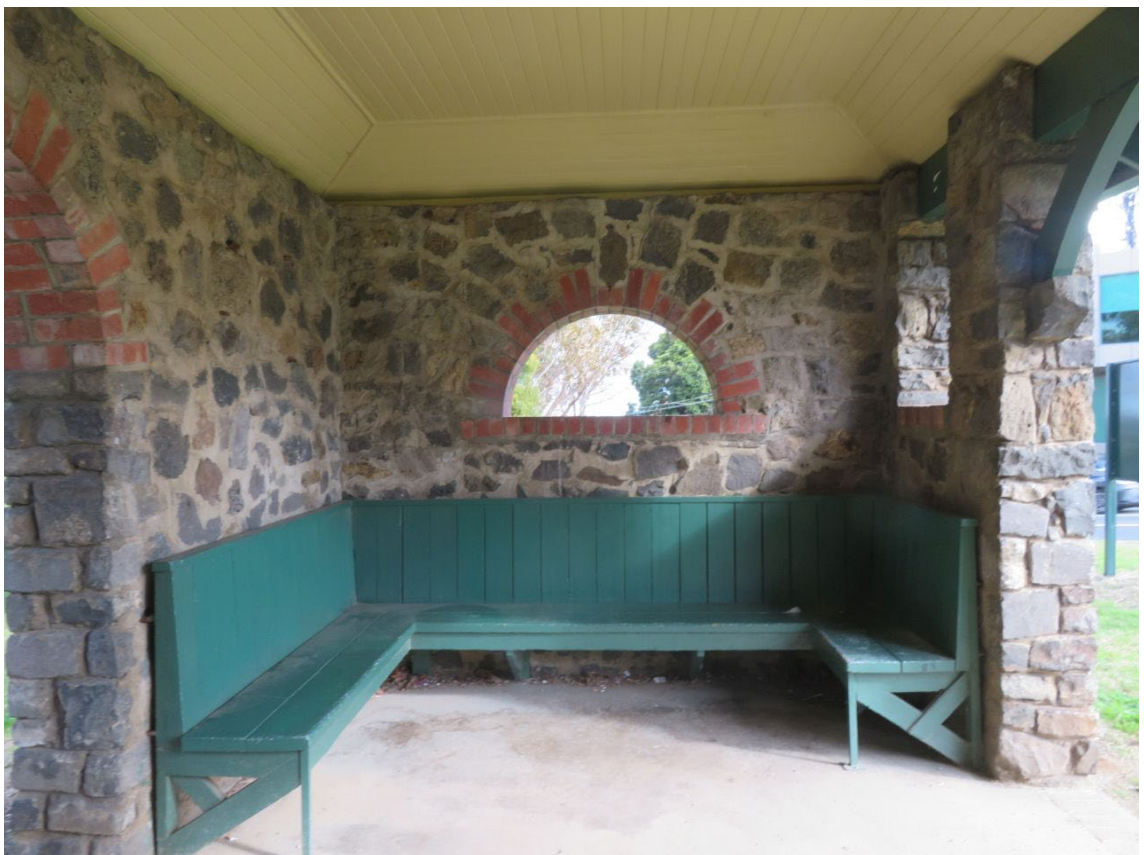
Figure 50 Seating inside the Tram Waiting Shelter at the corner of Warrigal and Riversdale roads
