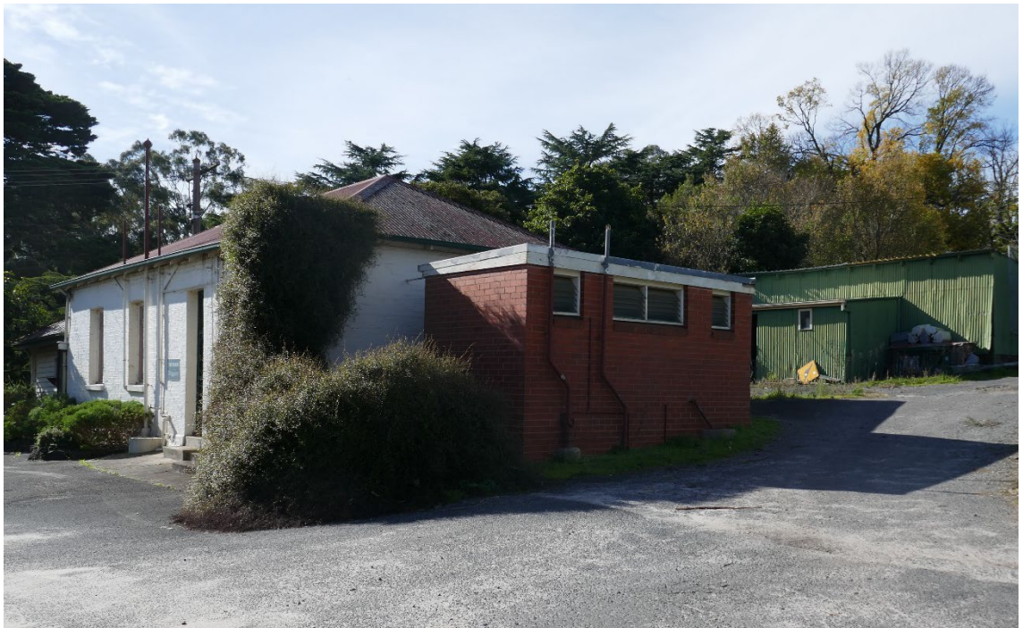
Figure 30 Addition to rear (west) of the Stables
