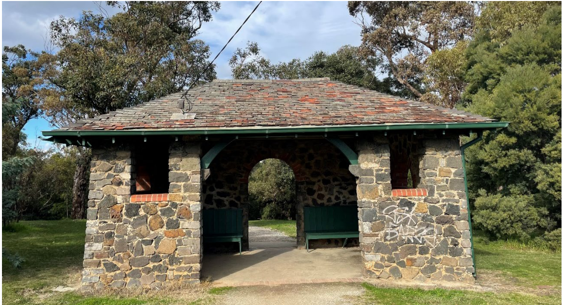
Figure 49 North-west elevation of the Tram Waiting Shelter at the corner of Warrigal and Riversdale roads
