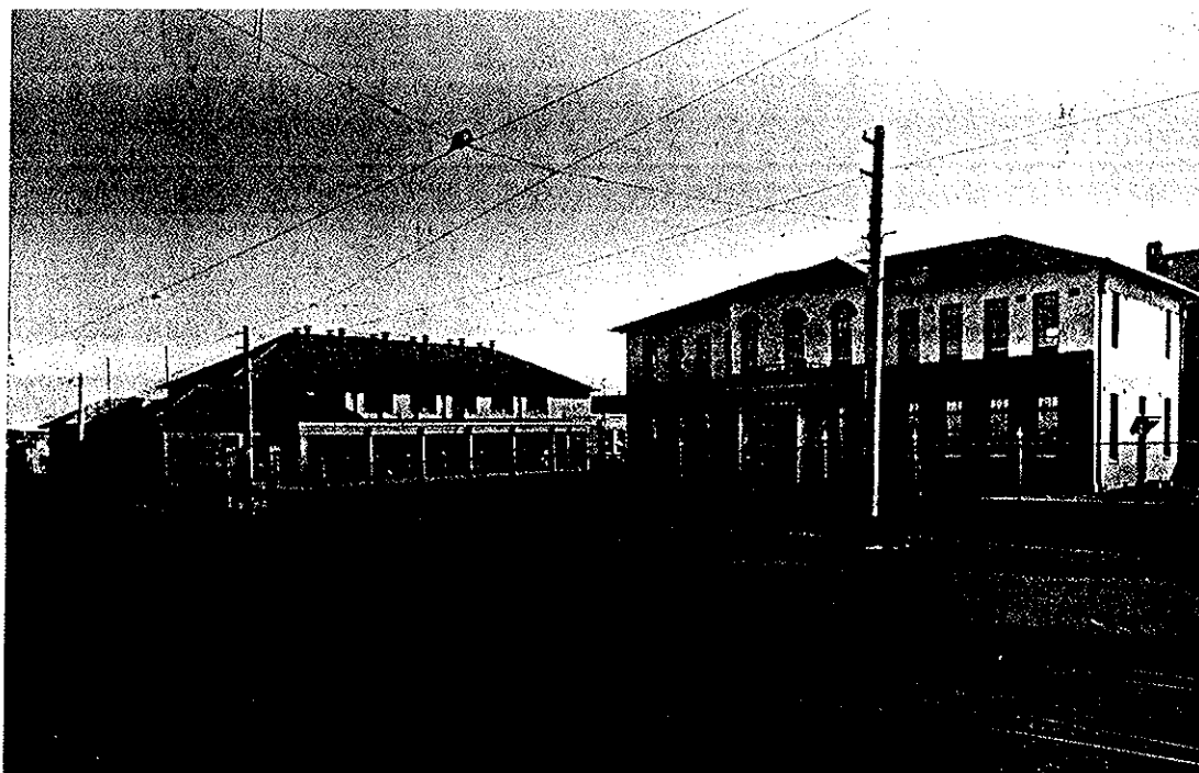
Figure 14 Mess Room and Offices, Preston Workshops. Source: Tramways Museum Society Collection.
