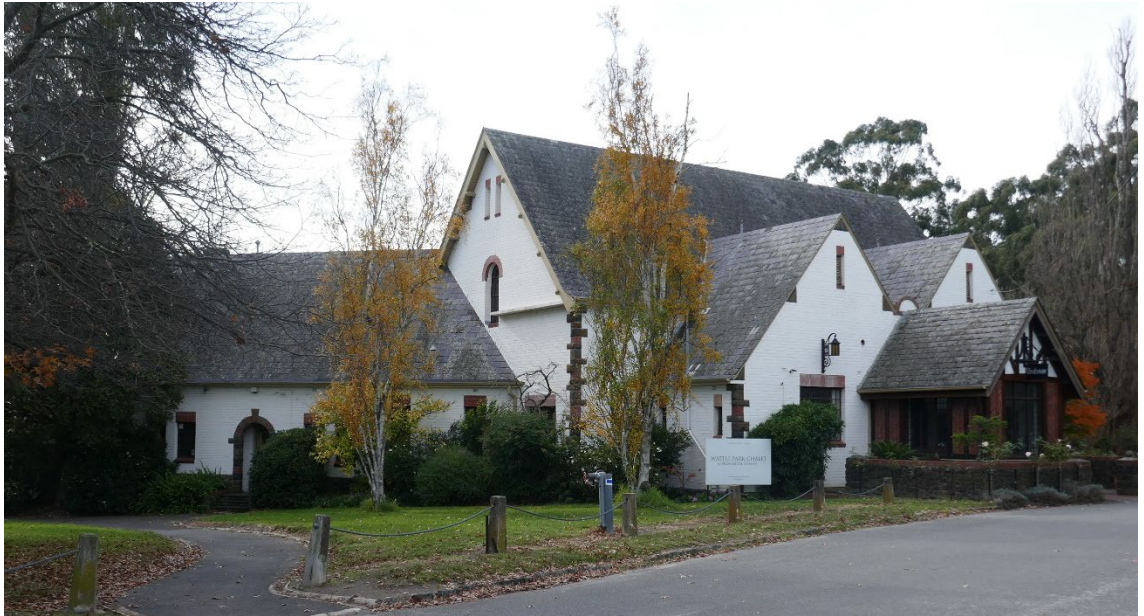
Figure 37 The Chalet, view looking north-east
