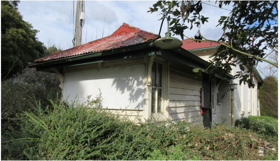
Figure 53 The Curator' Office: west (right) and north (left) elevations, with the Stables visible at rear
